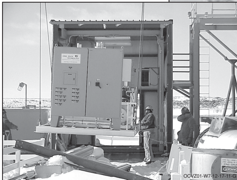
At the Radioactive Waste Management Complex workers install part of a system that is being used to remove underground organic contaminants.
