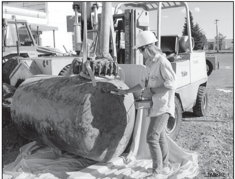
A radiation control technician checks a tank removed from the ground at the Test Reactor Area for any remaining contamination.
