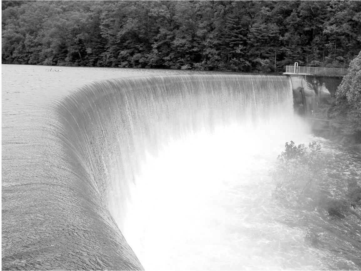
Lake Logan dam, North Carolina.
