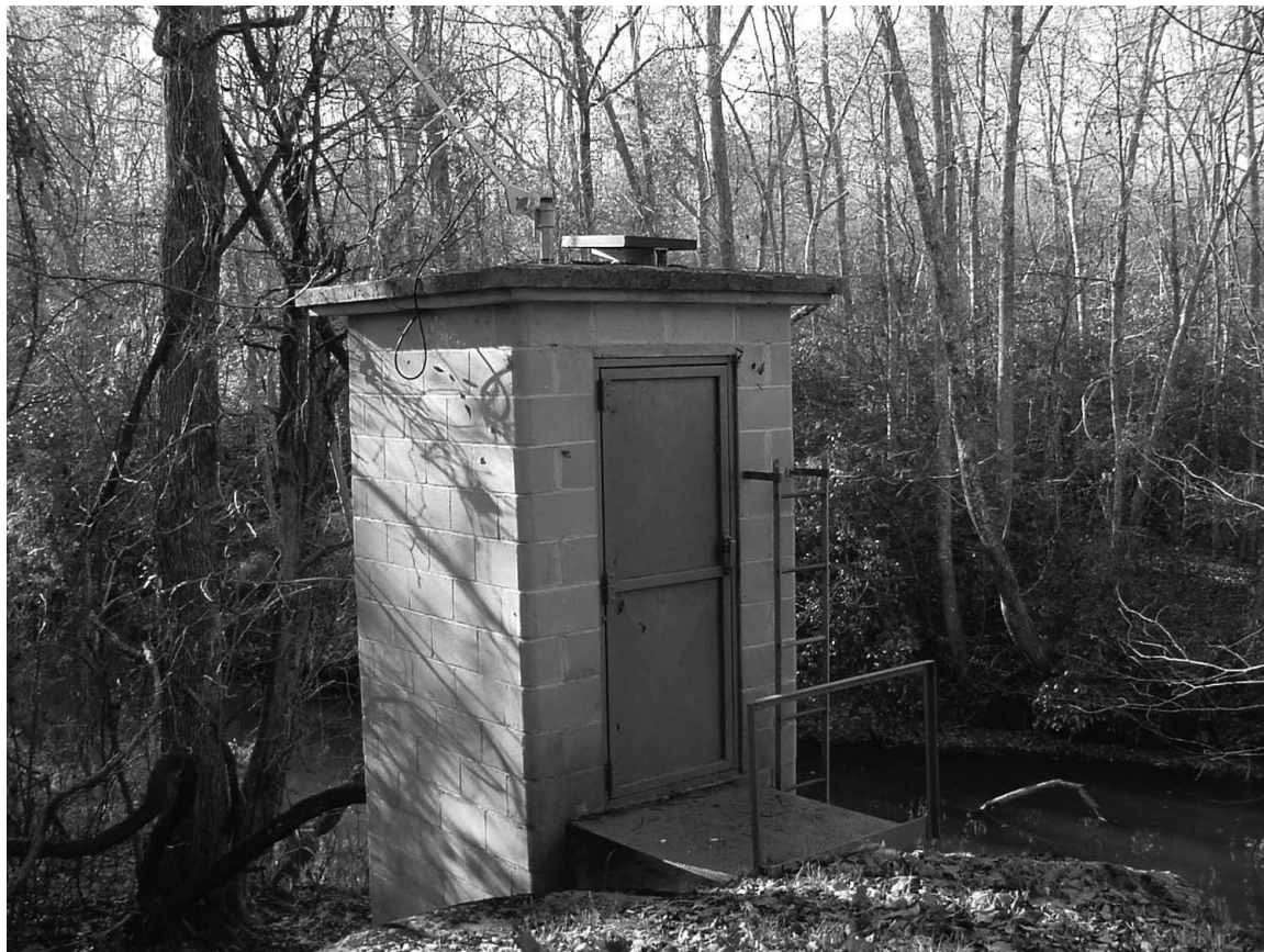
Gaging station at Long Creek near Bessemer City, North Carolina.
