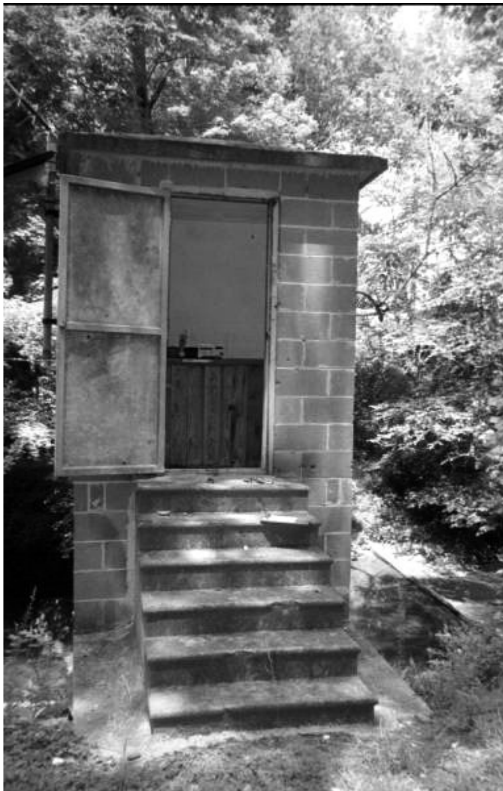
Gaging station at Mayo Creek near Bethel Hill, North Carolina.
