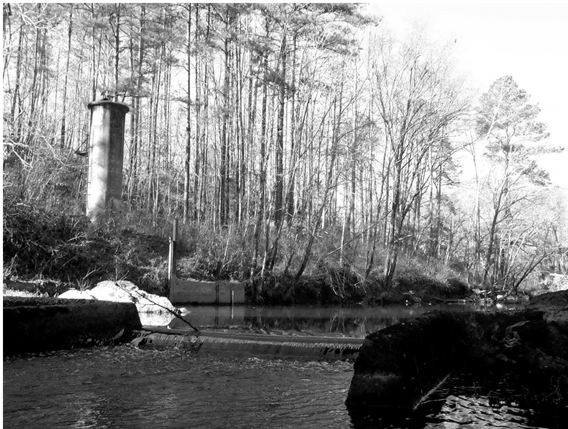
Gaging station and weir Tar River near Tar River, North Carolina.
