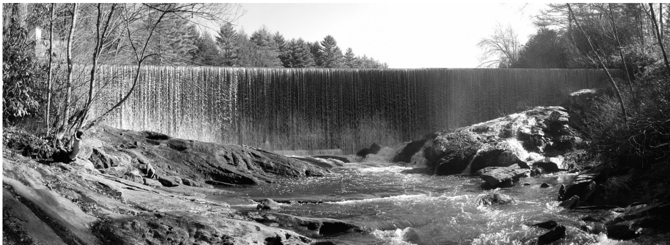
Flow over dam at Cullasaja River near Highlands, North Carolina.
