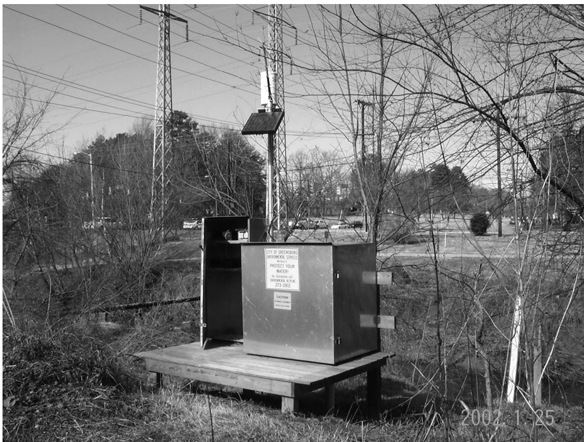
Gaging station at North Buffalo Creek at Westover Terrace at Greensboro, North Carolina.
