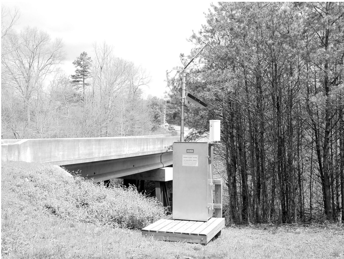
Gaging station at Second Broad River near Logan, North Carolina.
