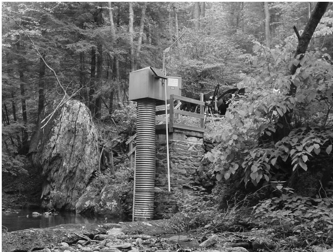
Gaging station at Beetree Creek near Swannanoa, North Carolina.
