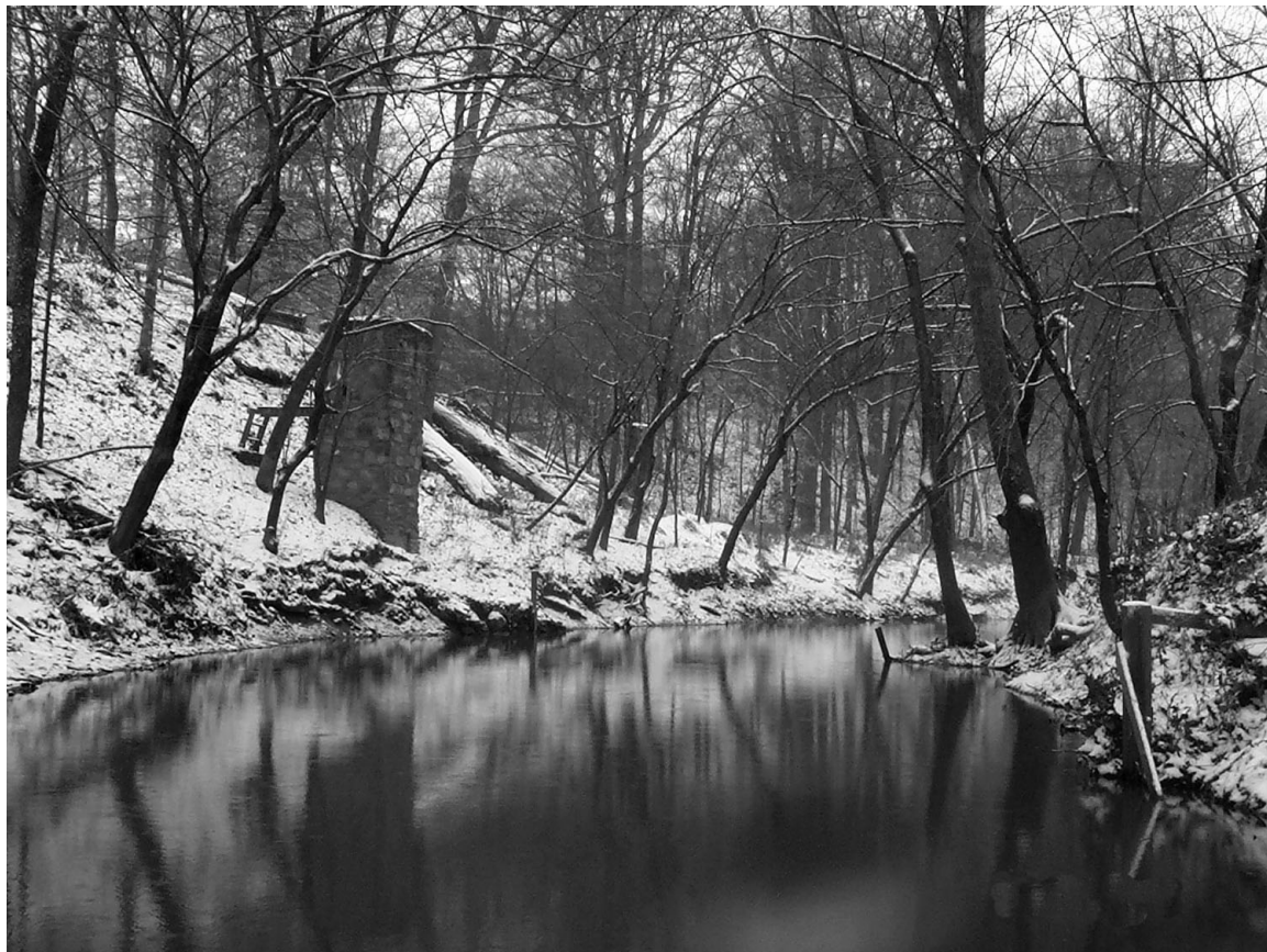
Old gaging structure at Eno River at Hillsborough, North Carolina.
