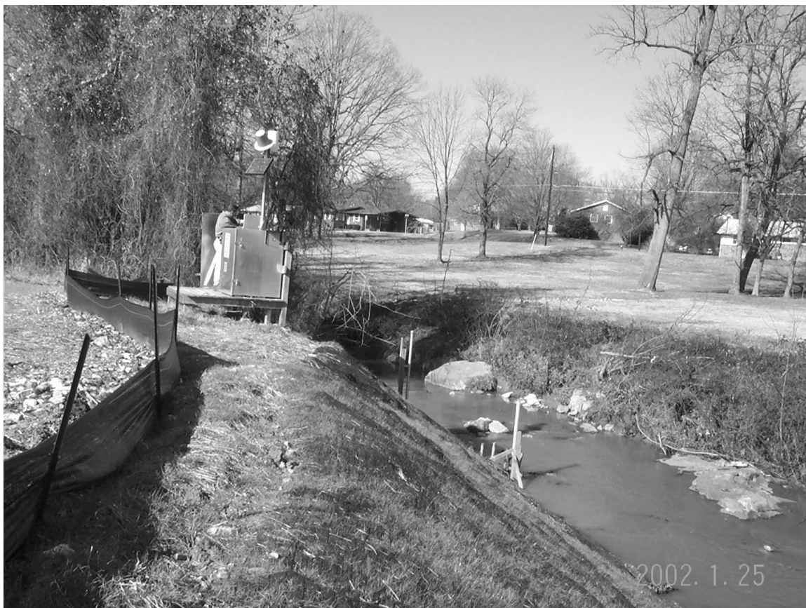
Gaging station at South Buffalo Creek near Pamona, North Carolina.
