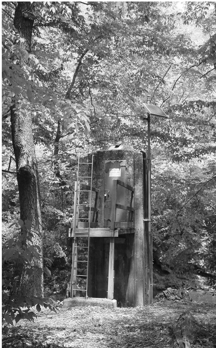
Gaging station at Mills River near Mills River, North Carolina.
