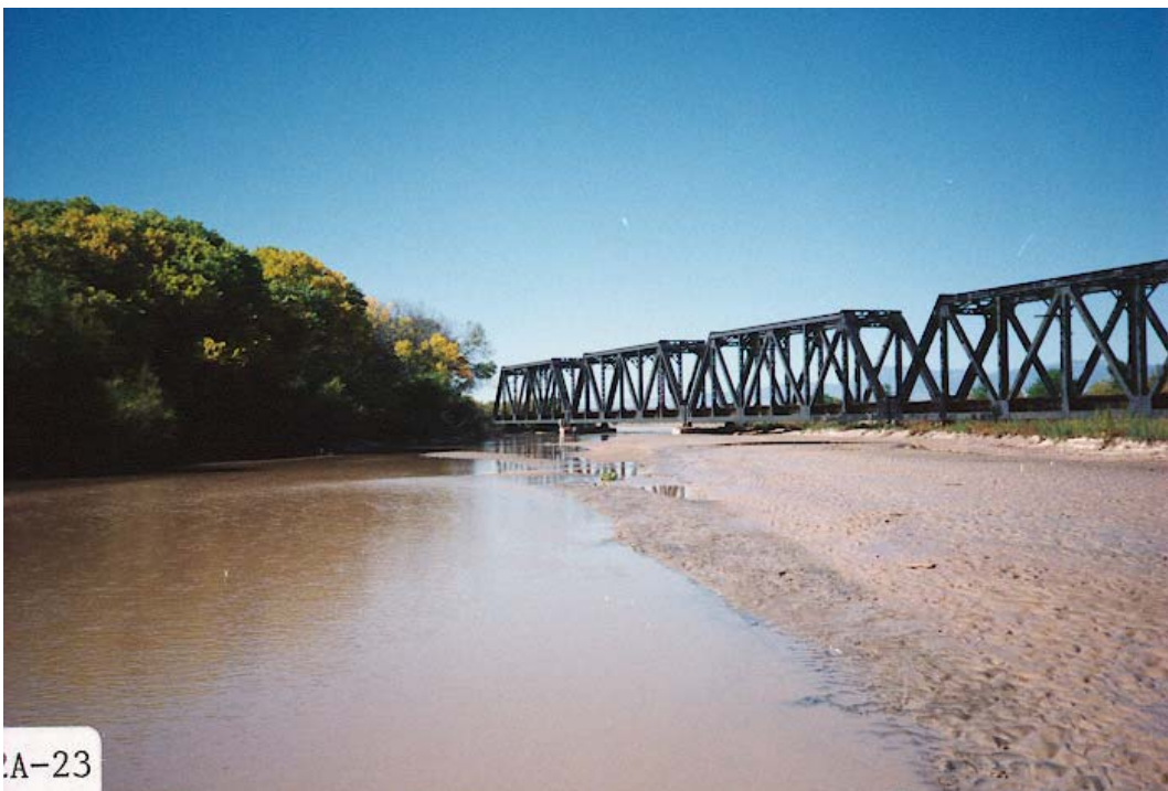
Photo 3.8 – The San Marcial Railroad Bridge (Reach 12)
