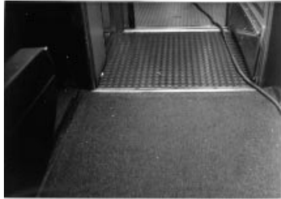
Figure 3-2. Carpet and Resilient Rubber Floor Covering
