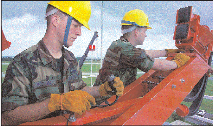
Airmen 1st Class Kenneth McClurg and Daniel Hickman replace the secondary radar antenna on Patrick Air Force Base's radar Tuesday. The 45th Space Communications Squadron, Federal Aviation Administration and Space Gateway Support will allow Daytona FAA controllers to route commercial air traffic through the area. (Photo by Jim Laviska)
