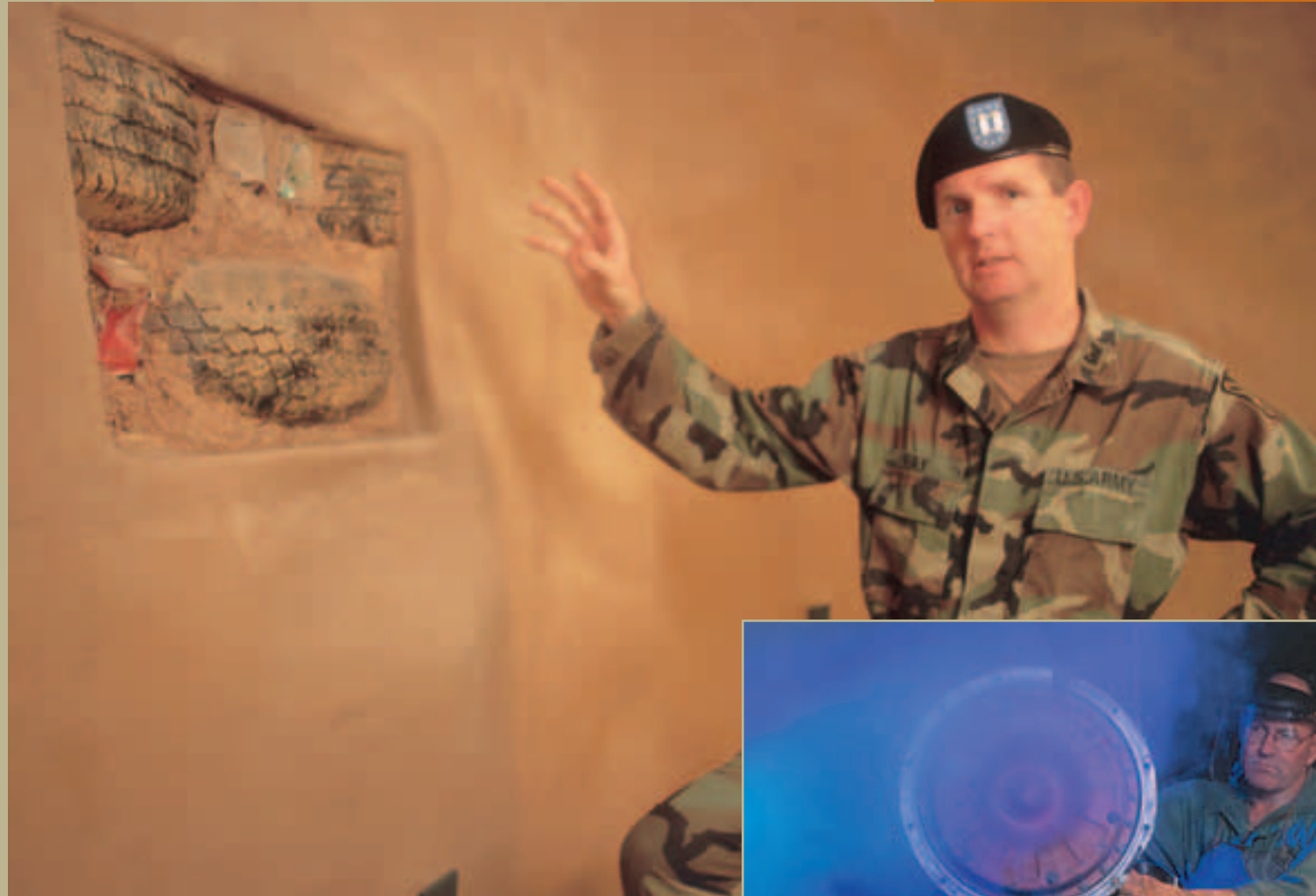
Capt. William Fay explains that recycled soda cans, used tires, mud and straw make up the structure of the “eco-building” at Papago Military Reservation in Phoenix, Arizona.
