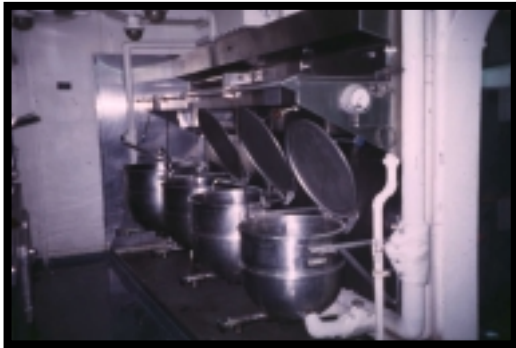
Fig. 2-6. Steam kettles.
