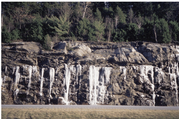
Ice formed on a road cut graphically illustrates the role of fractures in determining groundwater quantity. In this example, one near-horizontal fracture provides most of the water.
