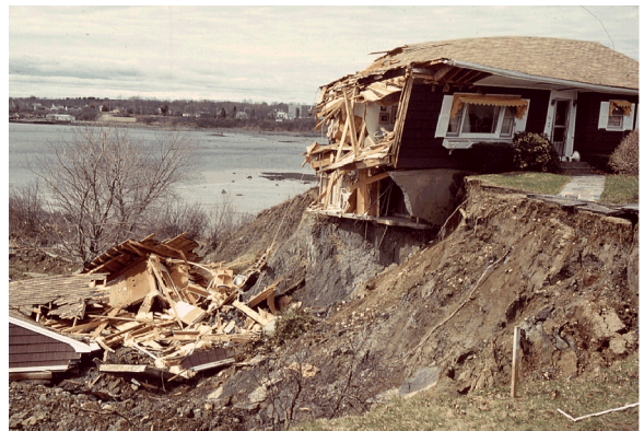
A large landslide in marine mud in Rockland in 1996 destroyed two homes.
