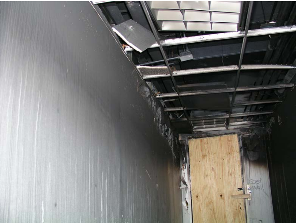
Figure 128. North corridor, looking towards the fire suite
