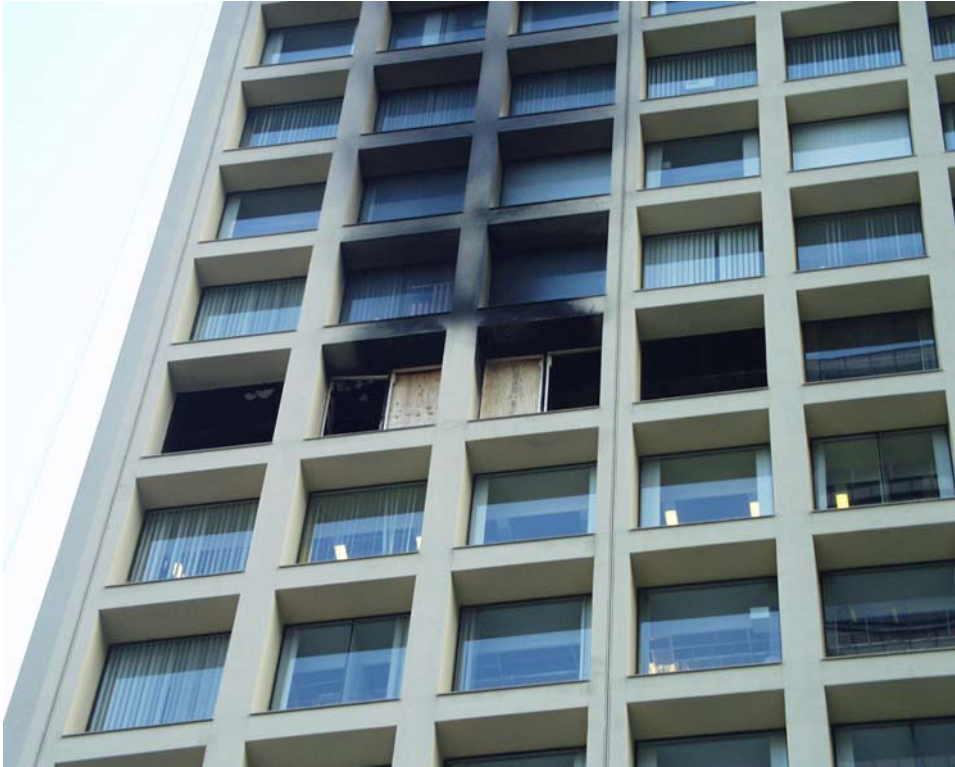
Figure 5. View of north side of the Cook County Administration Building
