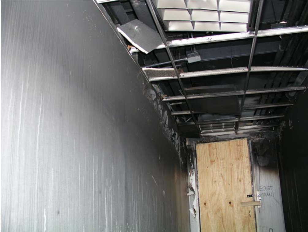
Figure 7. North corridor looking east to Suite 1240, main entry door
