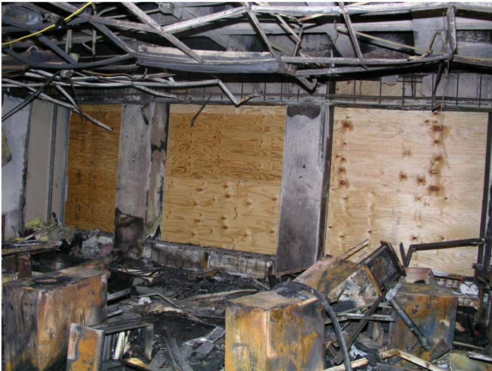
Figure 16. East northeast section of the open office portion of Suite 1240
