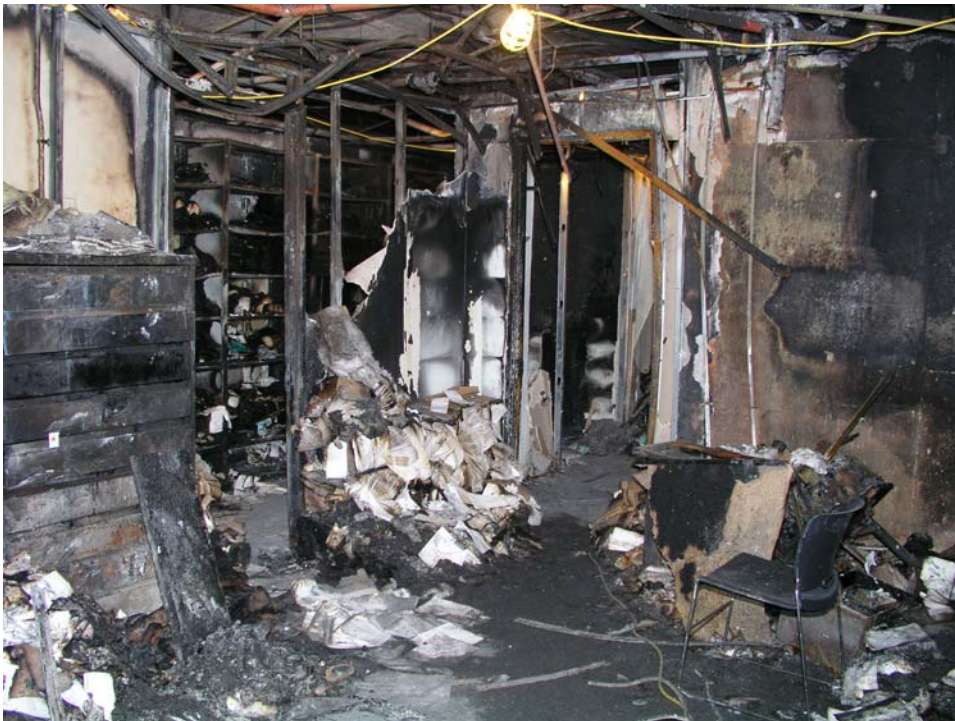
Figure 107. Material on floor in front of storage room
