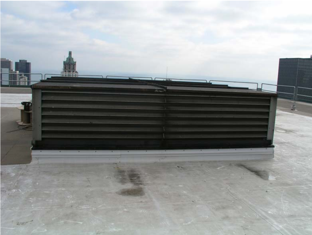
Figure 147. Top of smoke shaft on roof
