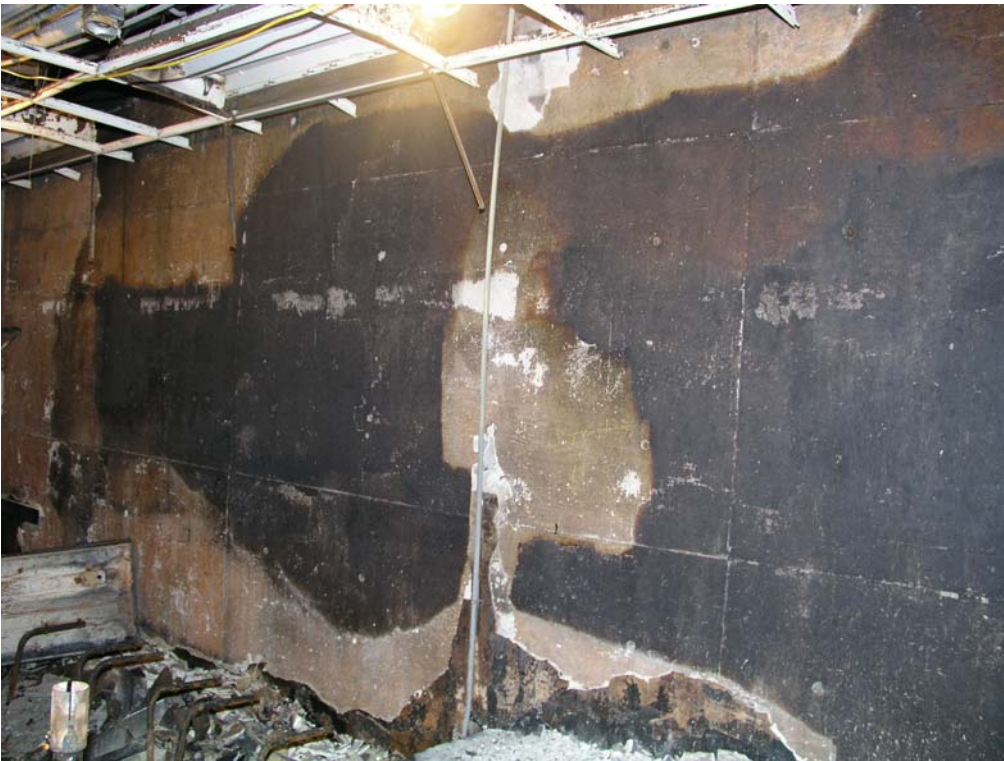
Figure 22. West wall of waiting area
