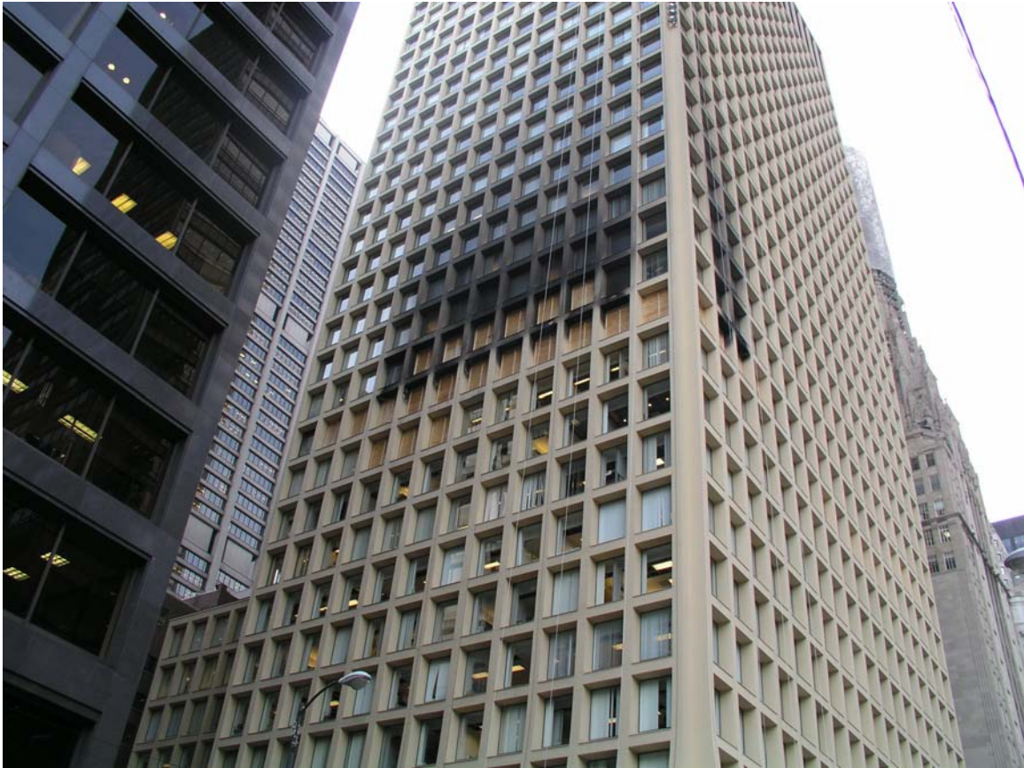
Figure 105. 69 West Washington Street – northeast corner
