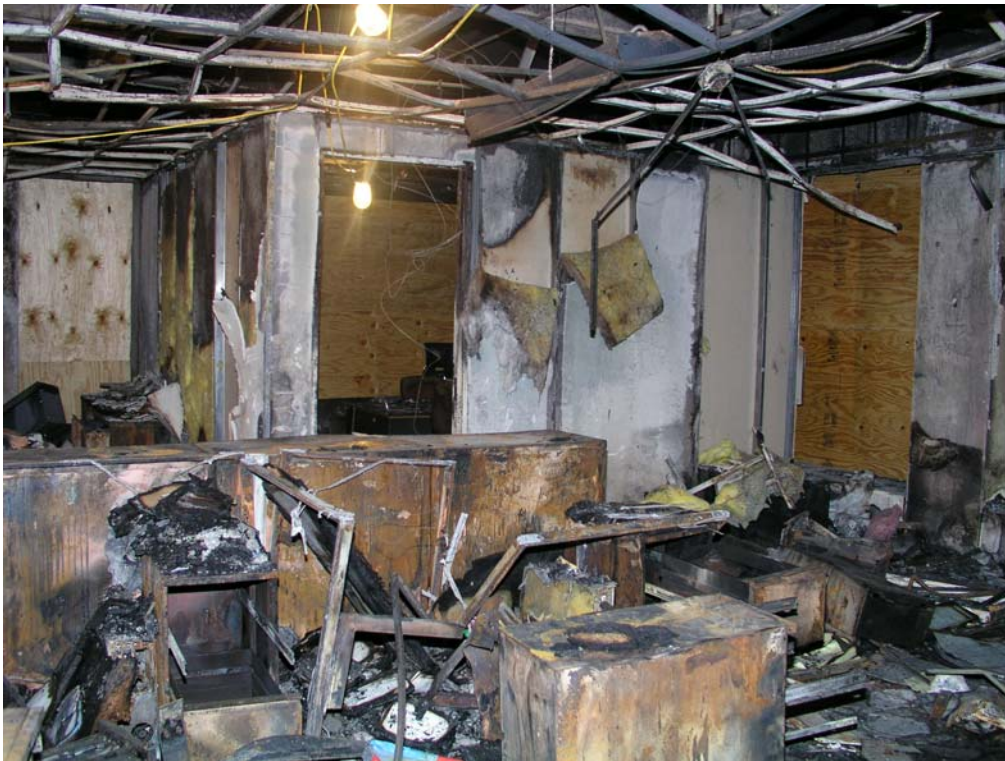
Figure 15. Northeast corner of Suite 1240
