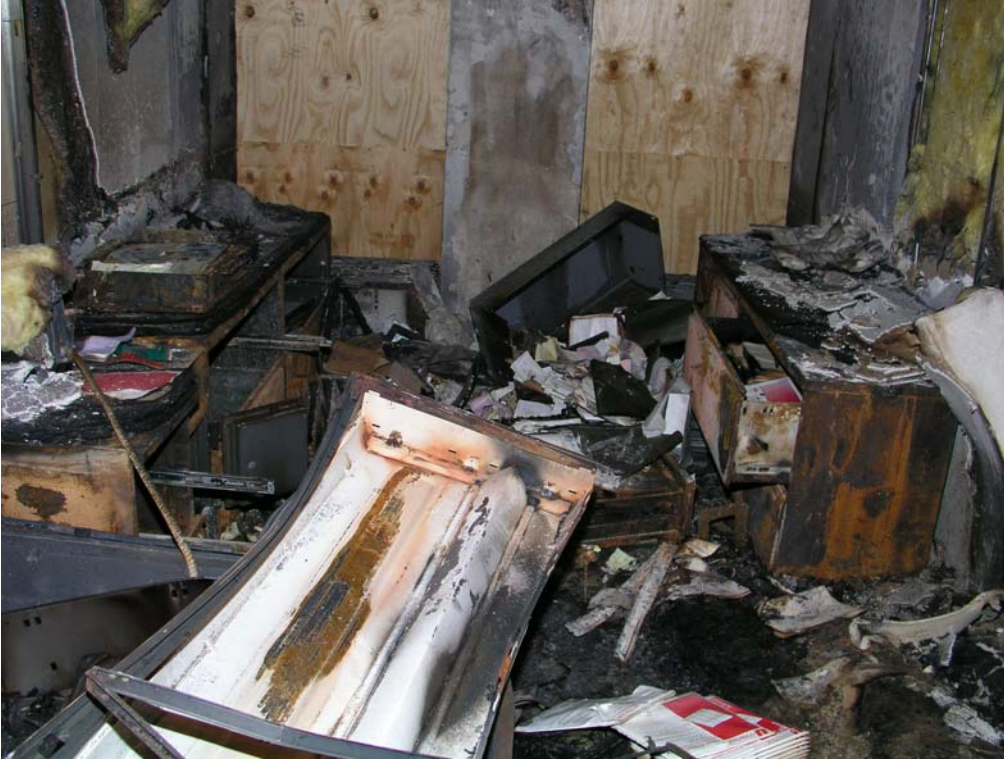
Figure 127. Fire suite, north end
