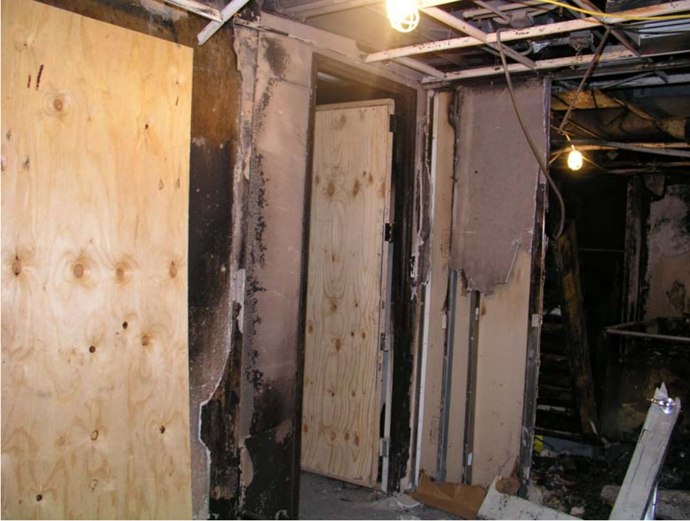
Figure 23. Main entry door from north corridor
