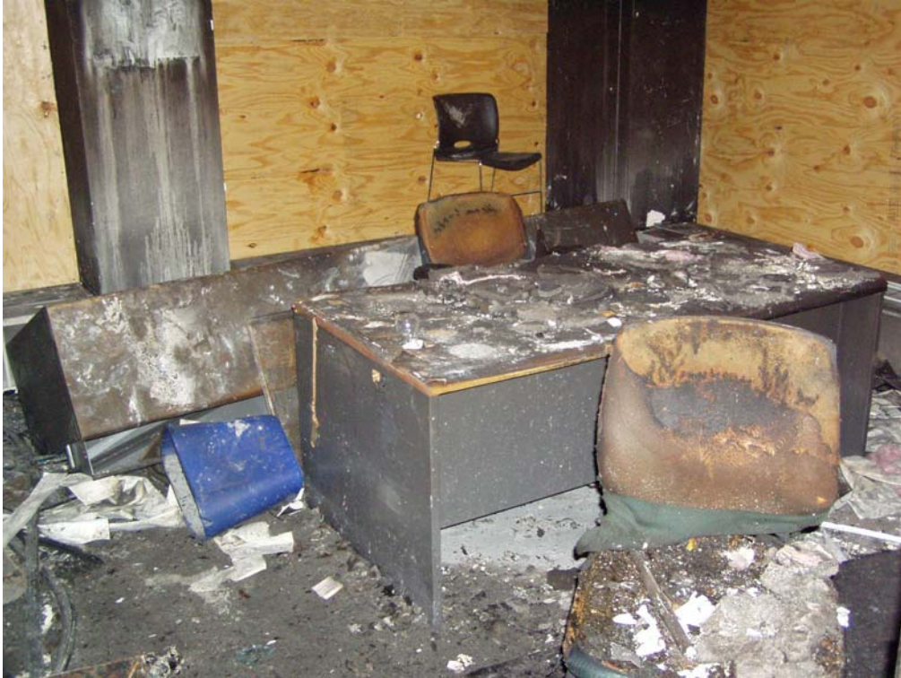
Figure 25. Northeast office in Suite 1240
