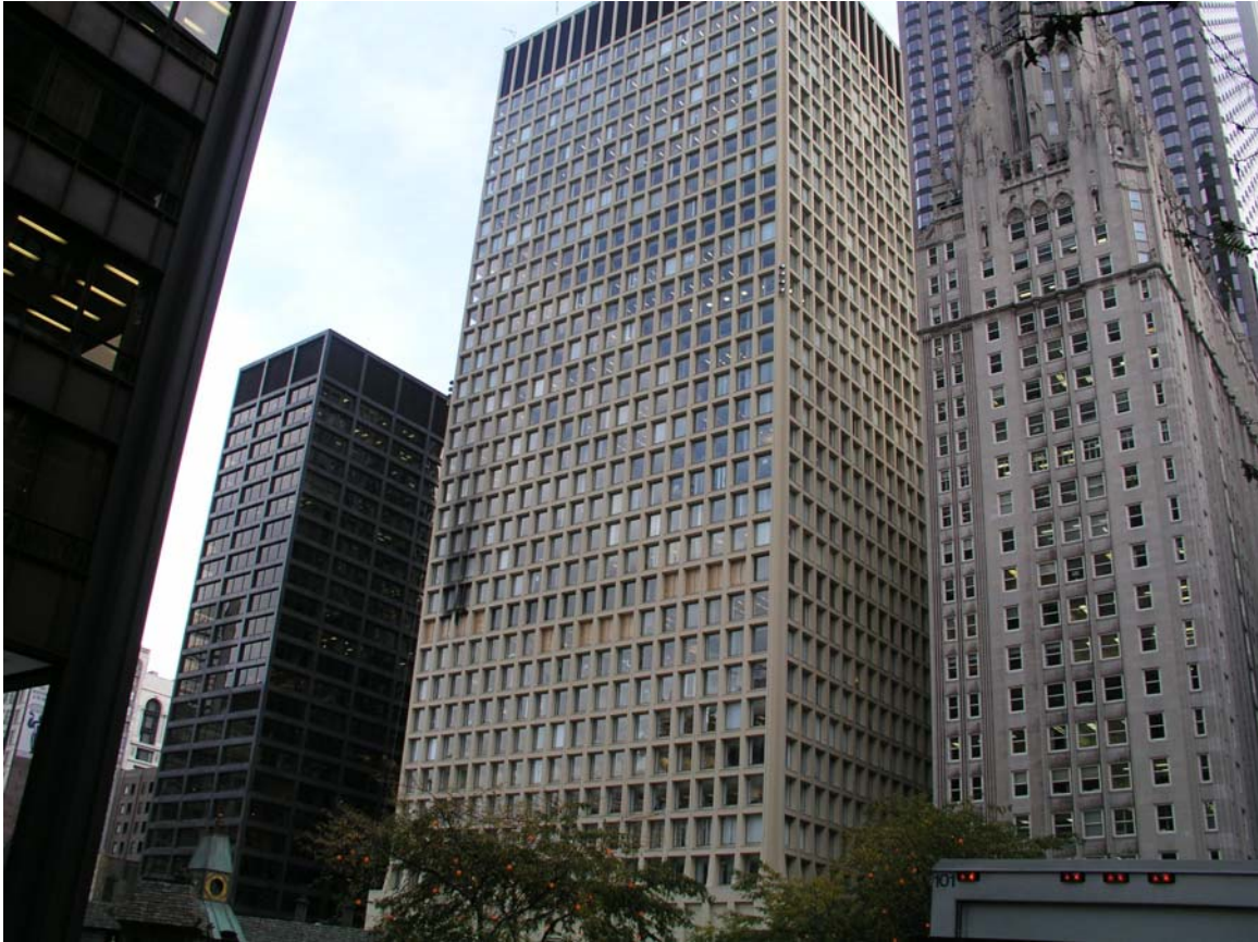
Figure 94. Cook County Administration Building, 69 West Washington Street – view from northwest
