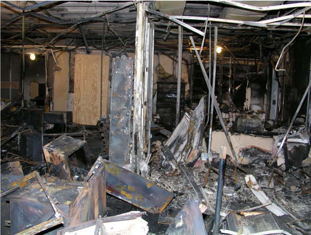
Figure 20. Looking south toward the storage room
