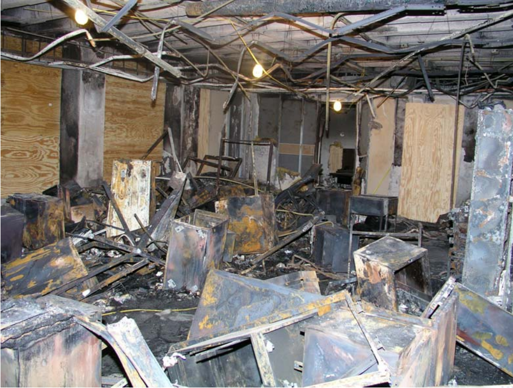
Figure 19. Looking toward the southeast corner of the Suite 1240
