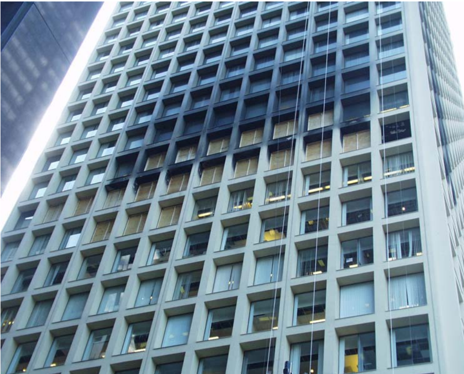
Figure 4. View of east side of the Cook County Administration Building
