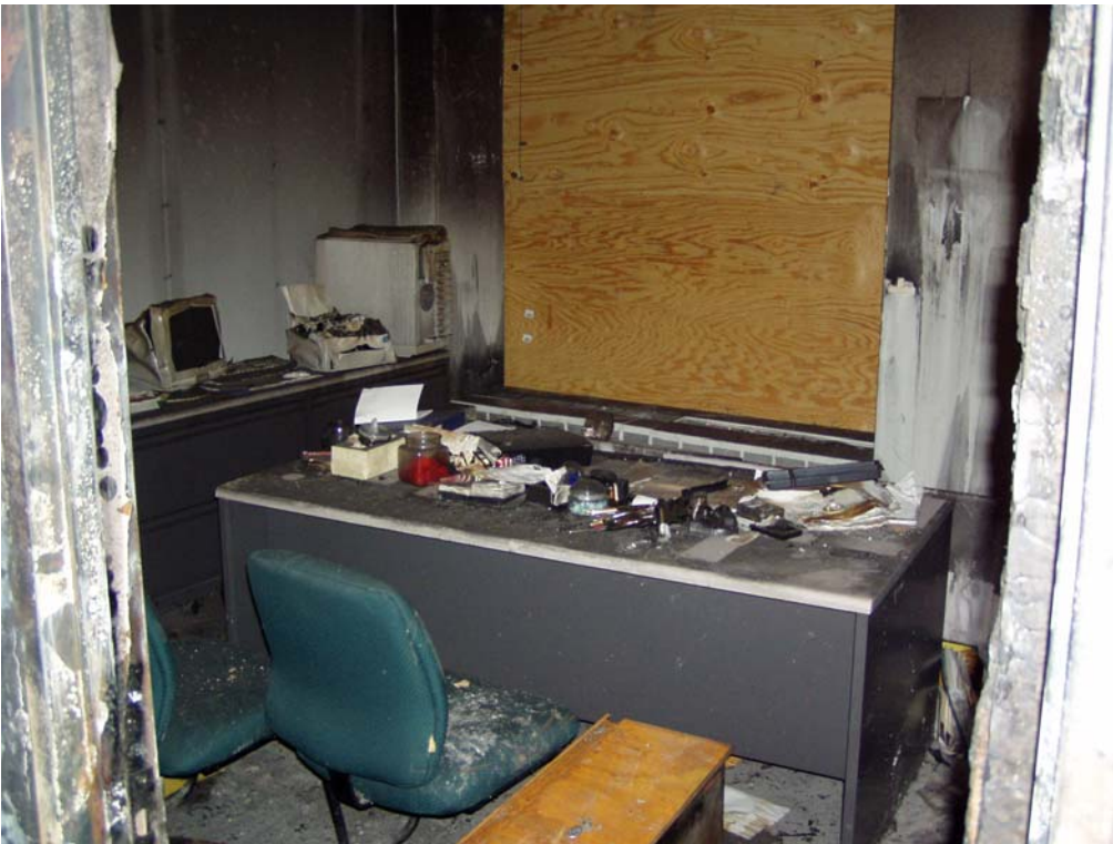
Figure 24. Northwest office in Suite 1240
