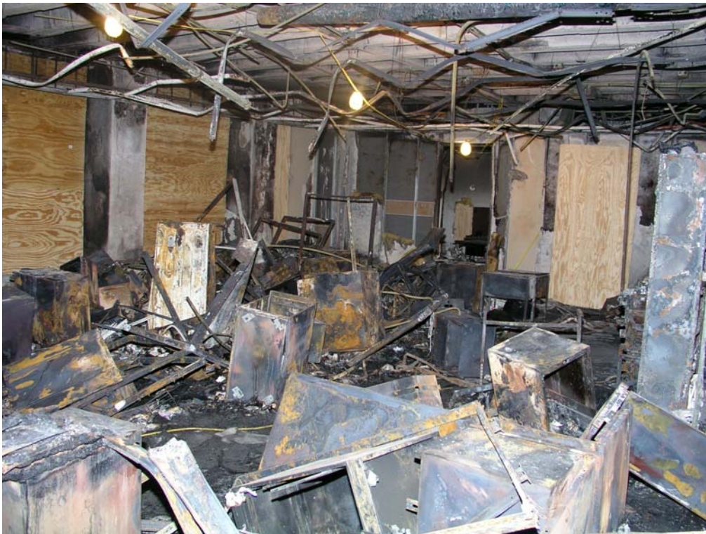
Figure 126. Fire suite, south end
