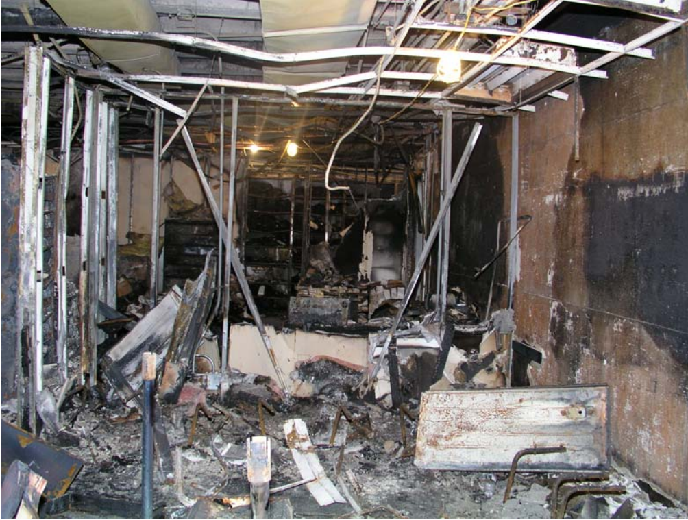
Figure 21. Looking south through the waiting area into the storage room
