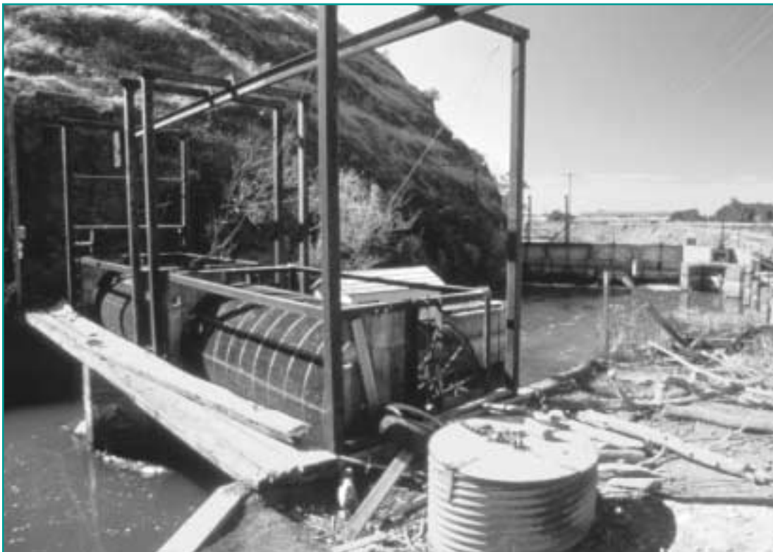
Screens are placed at the entrance to irrigation canals to keep fish from being diverted into channels that carry water away from the river.
