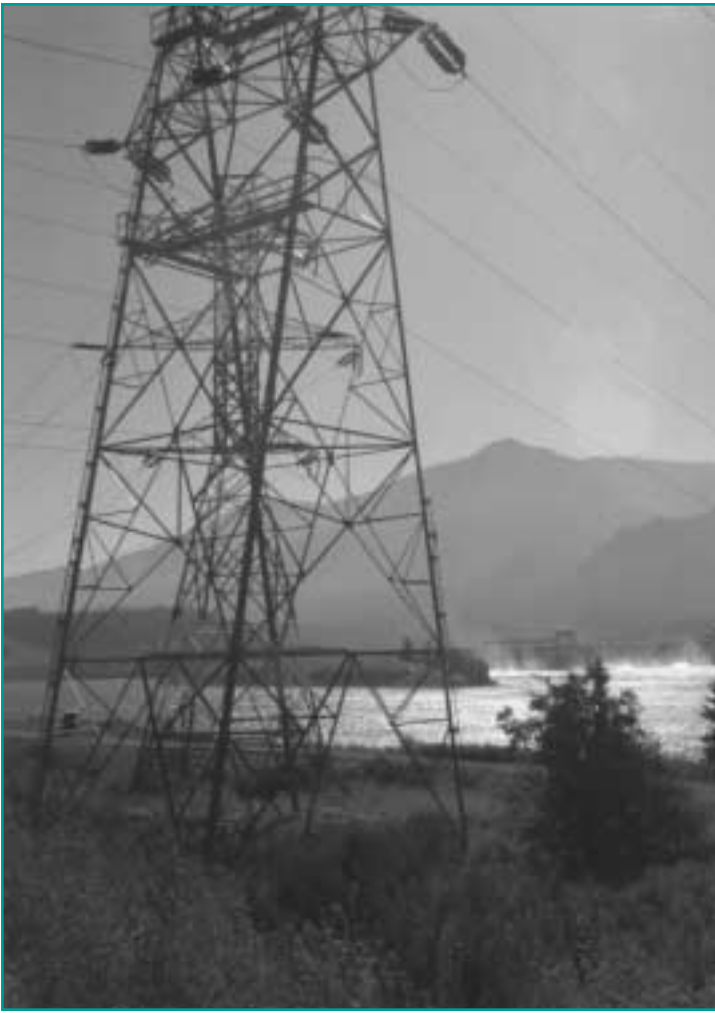
When runoff is high, BPA markets extra power to customers within and outside the region.
