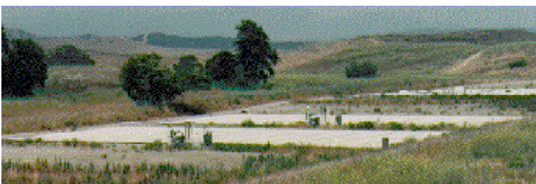
Innovative landfill capping technology.
