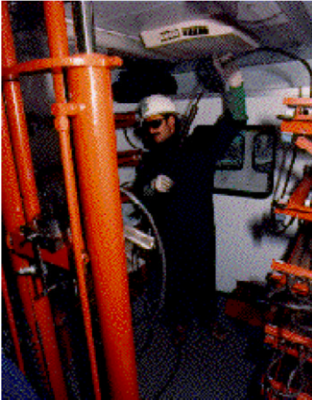
Push room operation.
