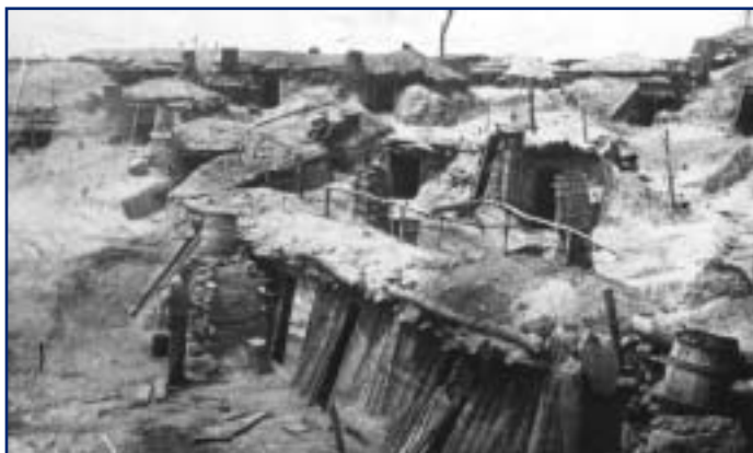
The Petersburg Trenches (Library of Congress)
