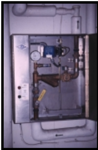
Fig. 2-10. Valve junction panel.
