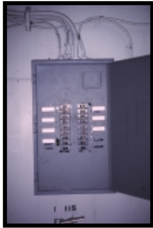
Fig. 2-9. Breaker panel.
