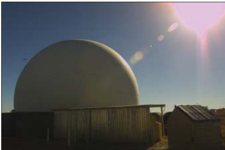
The Radome is a 60-foot diameter fiberglass-composite dome which is used for testing the AN/TPS 59. The dome has a maximum capacity of about 113097.34 units cubed, and allows the radar system to be fully opened fully inside of it.
