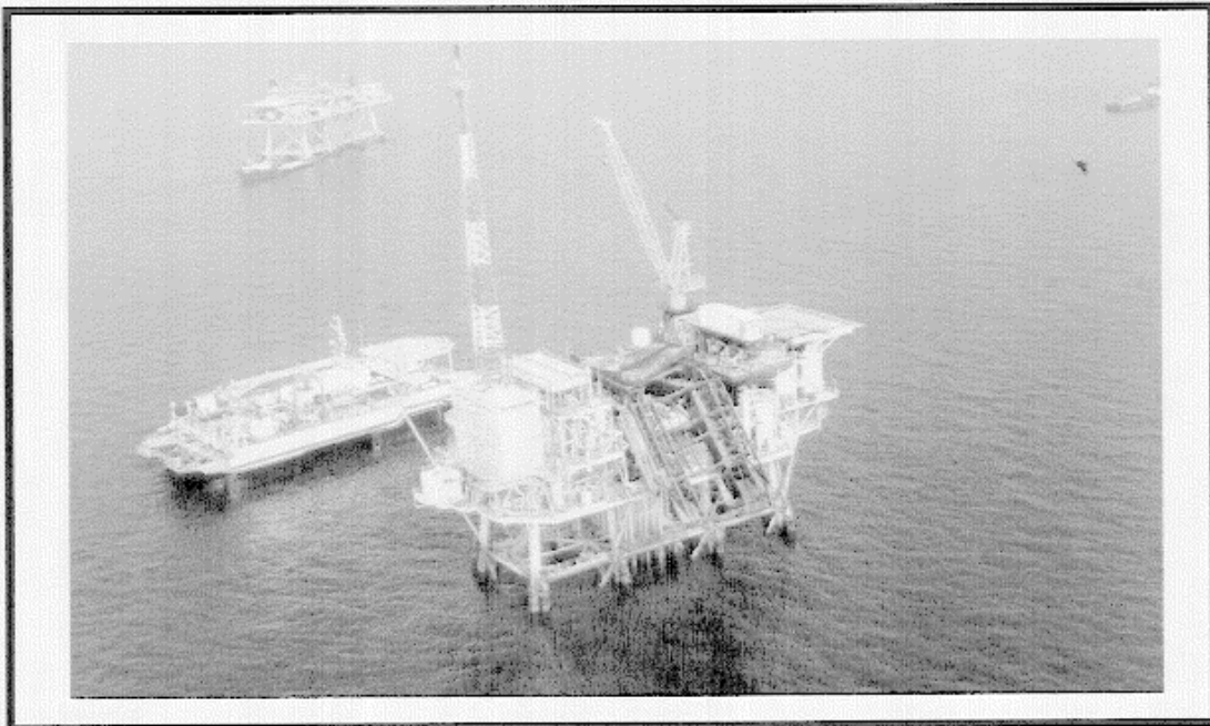
Photographs of Platform B After Accident
