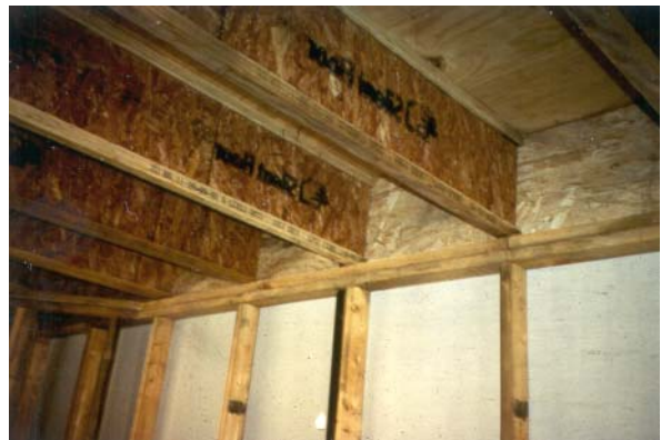
Fig. 18: In-line framing
