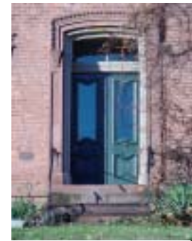
Fig. 9: Historic window and door
