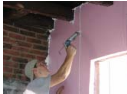
Fig. 25: Sealing joints between rigid insulation boards
