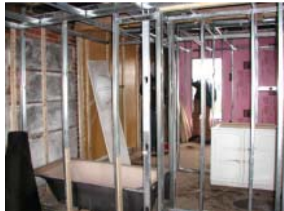
Fig. 20: Metal framing used for the interior partitions of this home
