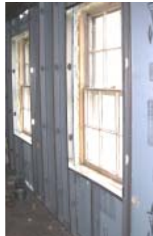
Fig. 25: Sealing joints between rigid insulation boards
