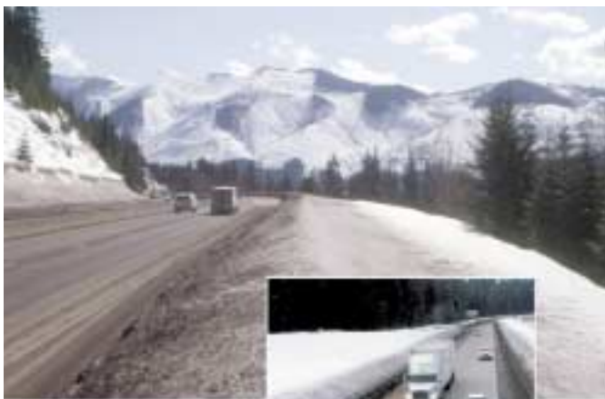
Interstate acts as a barrier to migration of some species, and poses visual management challenges.
