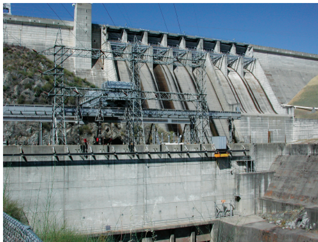
Figure 1: View of Folsom Dam.
