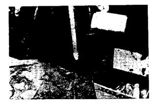
Filling soil in hole around the sleeve. (Sleeve temporarily extended to keep dirt out.) (13)
