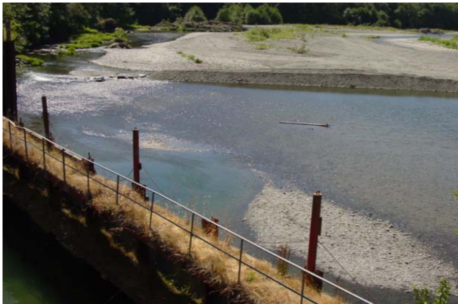
Completed Berm (connecting to the downstream grade-control weir, pictured)
