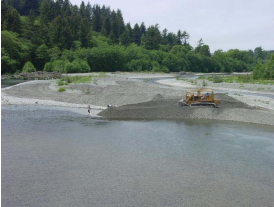
Berm During Construction (with federally-licensed biologist in the river protecting fish)
