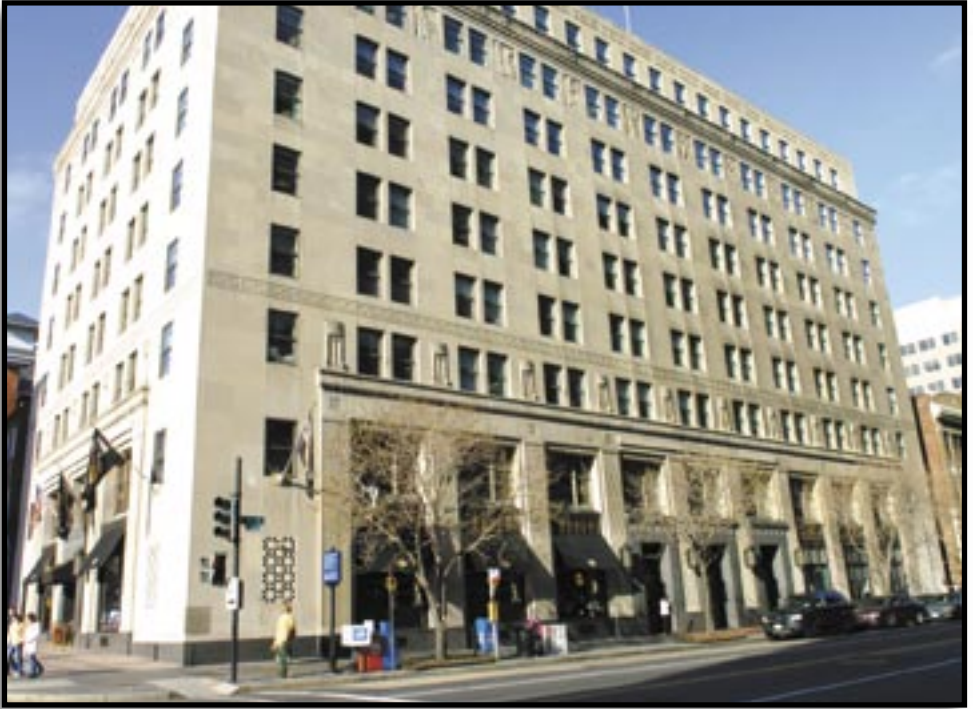
FEC Building in downtown Washington, D.C.
