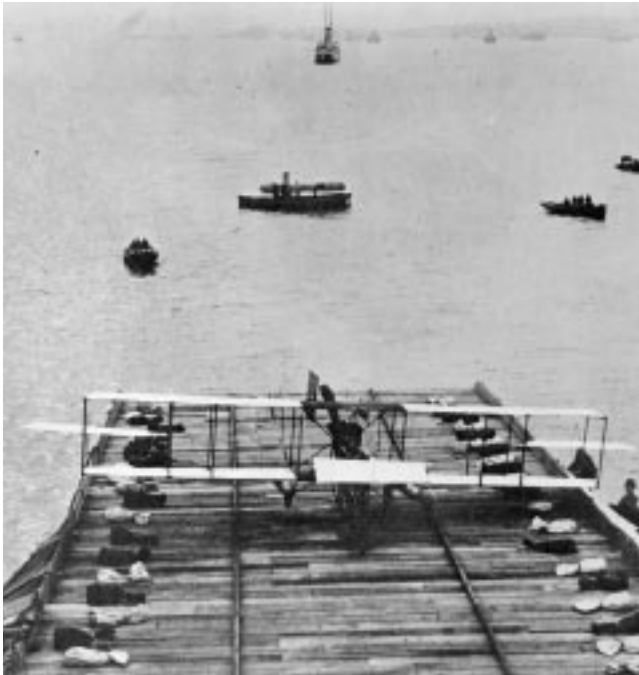
Sandbags, first arresting gear, halt Ely's plane 450108
