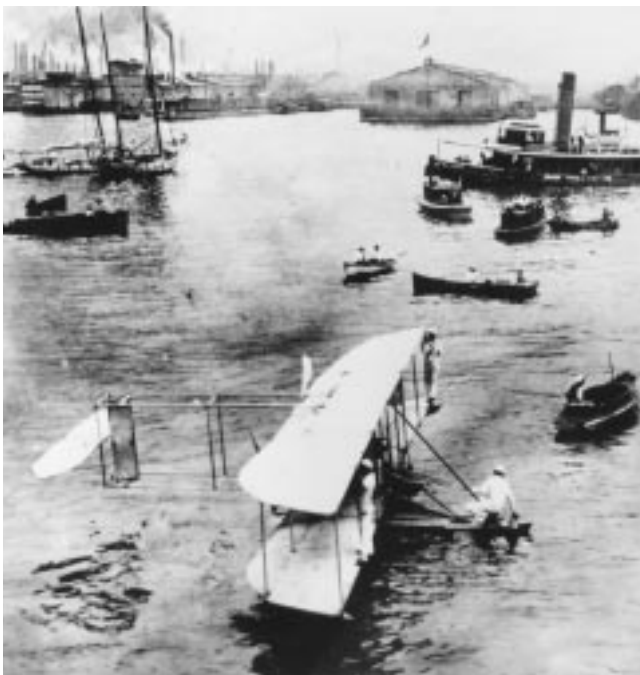
Navy Wright, B-1 after installation of pontoon 428225
