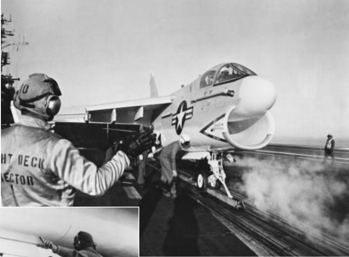
New way, A-7 launch with nose tow gear 119077
