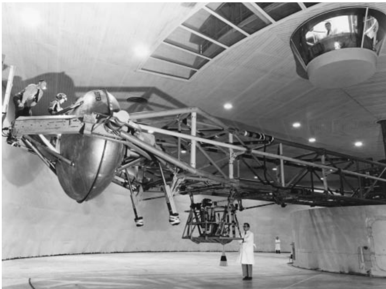
Human centrifuge used in study of space flight 1036457
