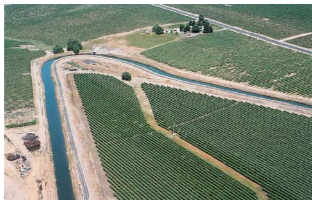
Pump station near drain at Snipes Road.
