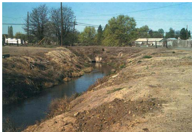
Granger Drain at Granger looking upstream.
