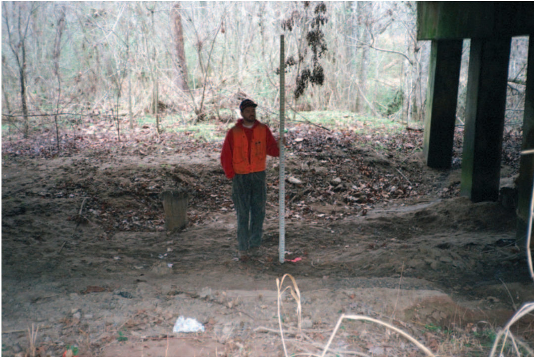
Figure 99. Example of shallow clear-water contraction scour at Structure 464032200300 on S.C. Route 322, crossing Fishing Creek in York County, South Carolina. (Photograph by the South Carolina District, U.S. Geological Survey, January 28, 1997.)
