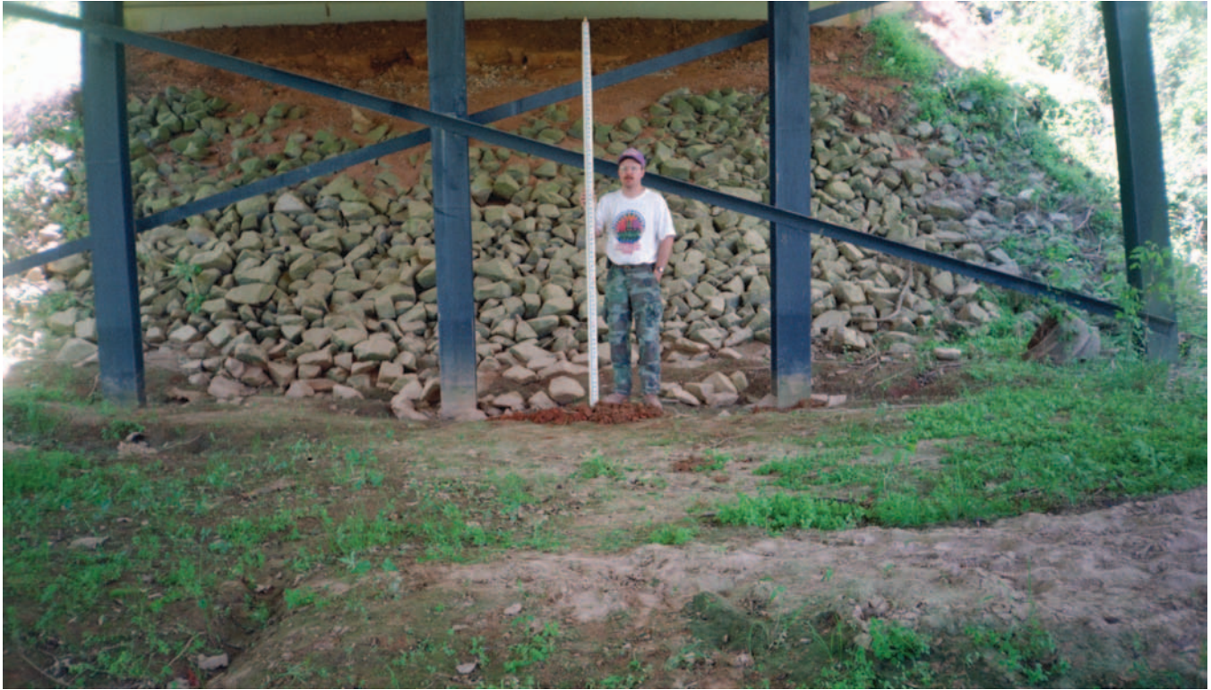
Figure 31. Spill-through abutment at structure 307011200100 on Road S-112, crossing the Enoree River in Laurens County, South Carolina. (Photograph by the South Carolina District, U.S. Geological Survey, April 2, 1997.)
