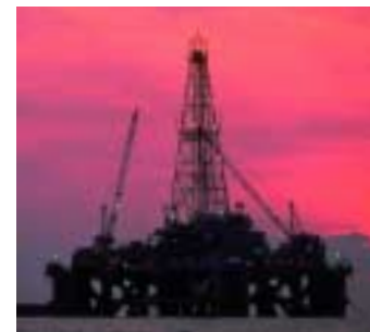
MMS's fleet of 13 helicopters and 55 inspectors reviews the operations of the 3,900 platforms in the Gulf of Mexico. When problems are discovered, we issue safety alerts to give all operators and training centers a heads up.
