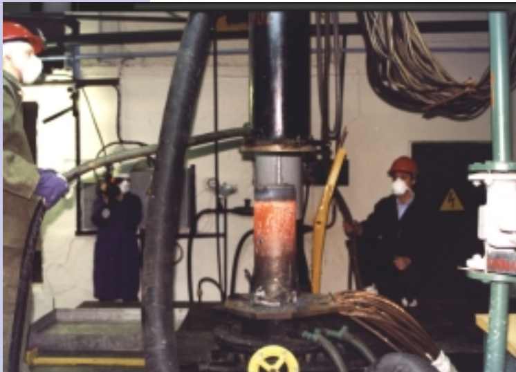
ElectroSlag Remelting (ESR) process for radioactive decontamination of stainless steel scrap for metal recycle. [see Project #60363]
