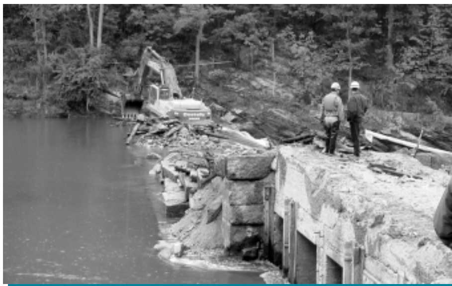
The Smelt Hill Dam in New Hampshire is breached during removal.
