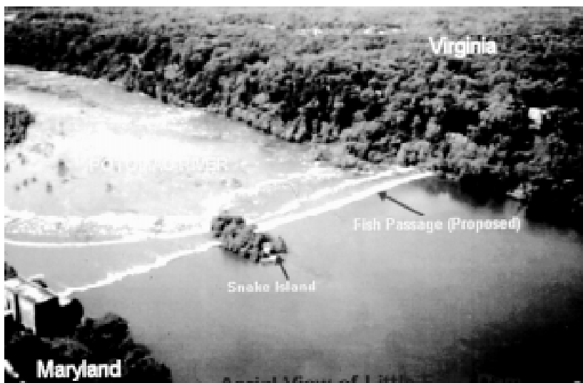
Little Falls Dam on the Potomac River.
