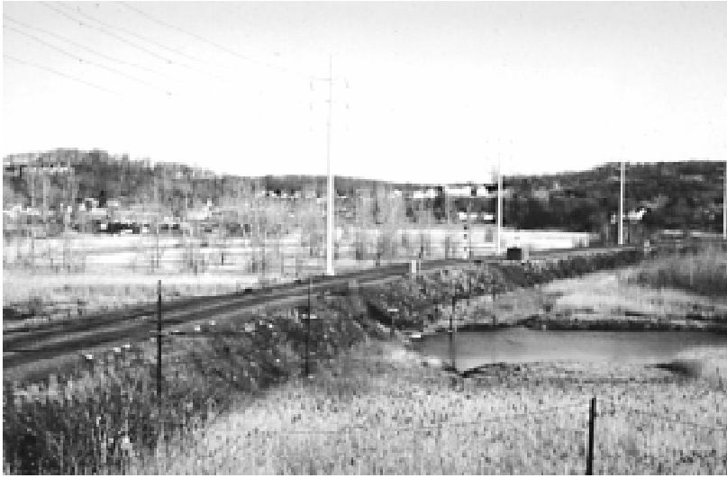
Restricted tidal flow as a result of railbeds in the Northeast Corridor, CT.
