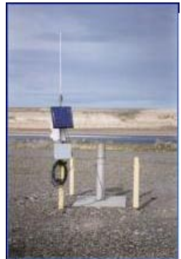
Groundwater monitoring well along river
