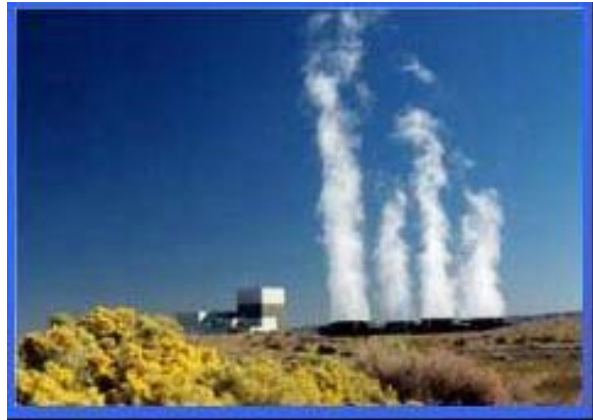
Energy Northwest Columbia Generating Station
