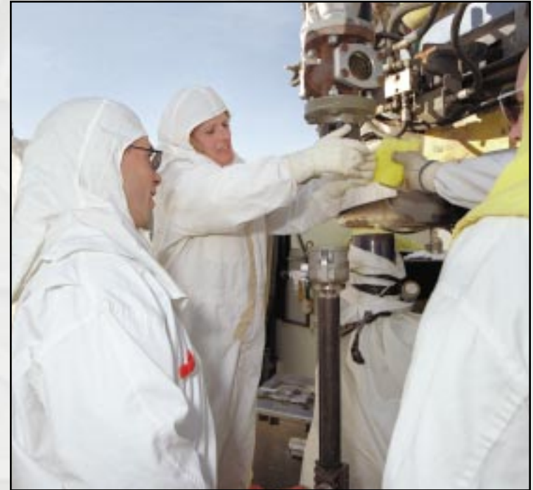
Workers obtain a sample of gases retained inside Tank SY-101.
