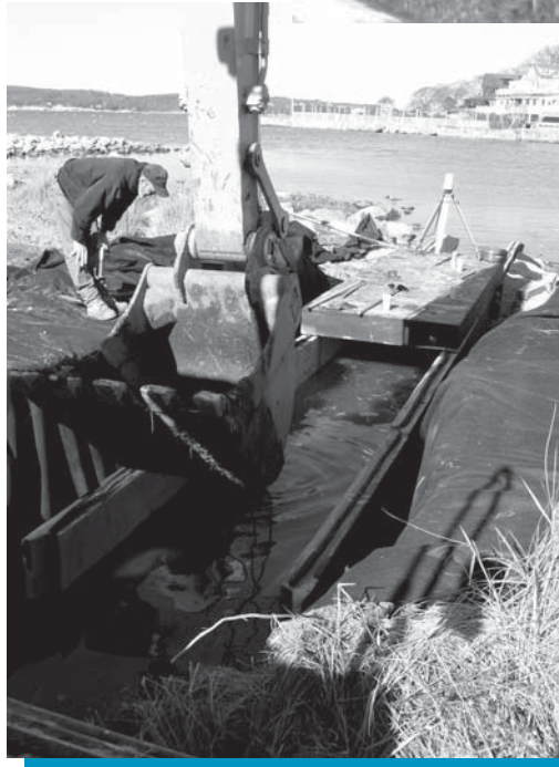
The Massachusetts CWRP culvert project will strengthen the natural ecosystem.
