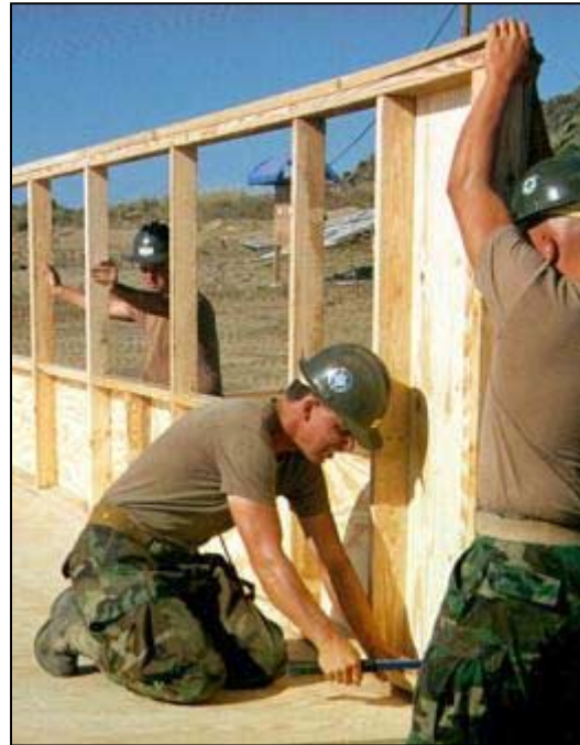
Photo 5. Army Vertical Construction
