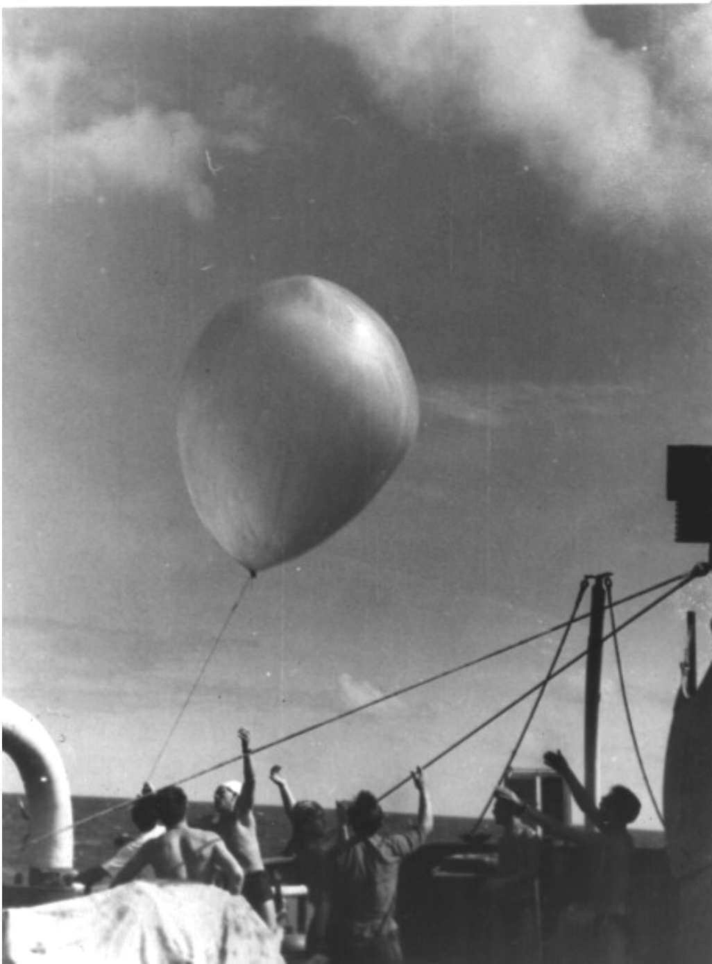
Launching a radiosonde from a research vessel
