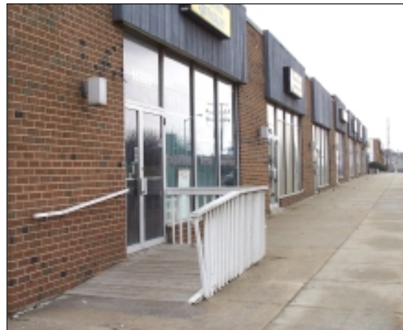
City zoning policies were changed to permit this business to install a ramp at its entrance.
