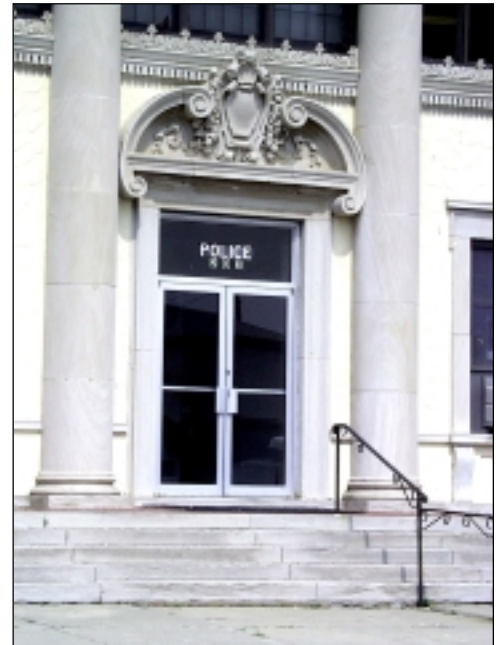
Cities must remove barriers or provide alternative access to programs and services in existing facilities.
