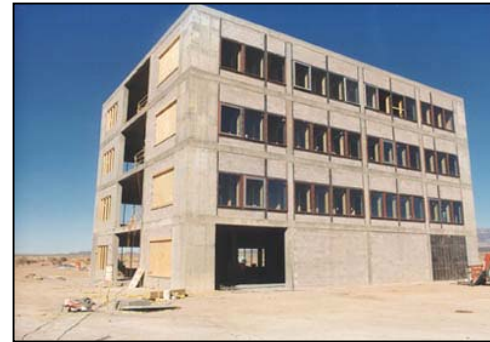
Component Test Structure-1 (CTS-1)
