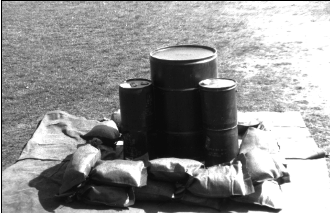
Figure 1: Secondary containment illustrated above consists of a tarp and sand bag perimeter large enough to contain 10% of the overall volume or 100% of the volume of the largest container stored. This is designed to protect human health and the environment in the event of a leak or spill. To maximize containment, the underlying tarp can be wrapped around the outside perimeter of the sand bags and folded back into the storage area.
