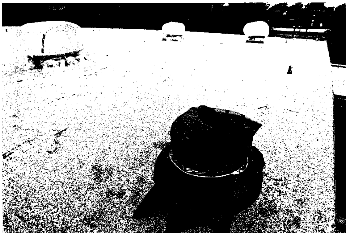
Figure 6. A Sealed Building Exhaust System.
