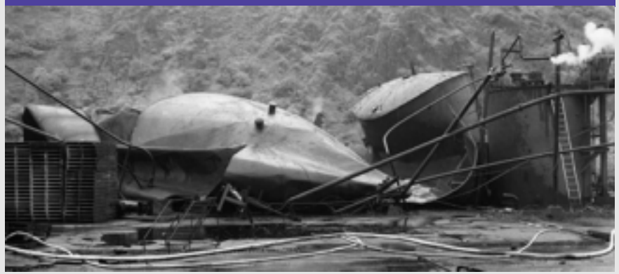
● Figure 8. WESTVACO paper mill tank failure.
