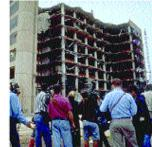
Protecting America's Infrastructure - Sandia is working to raise construction standards to produce structures that can better withstand a wide range of threats. In the Oklahoma City bombing, most of the victims were killed not by the blast but by the building when its nine floors collapsed like a house of
