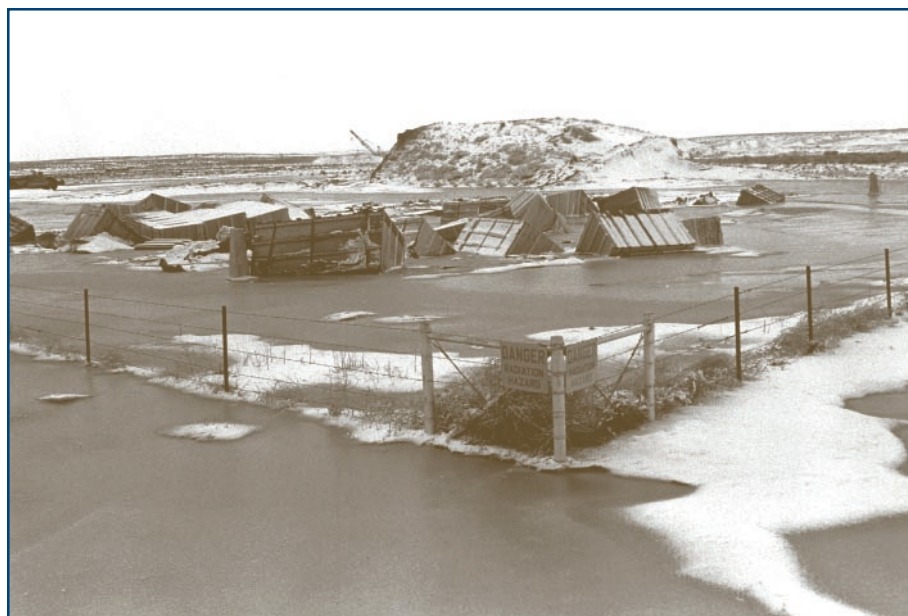
Figure 24. Water, flowing from the surrounding terrain (such as during this 1969 flood), has entered open excavations at the Radioactive Waste Management Complex and possibly leached contaminants from buried waste into the vadose zone. Dikes have been constructed to protect the complex from future floods.
