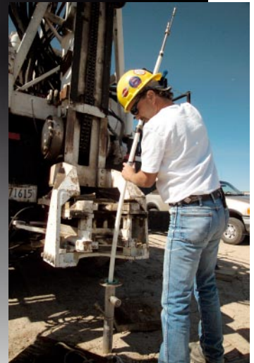
Installing an instrument into the probe casing is safe and easy.
