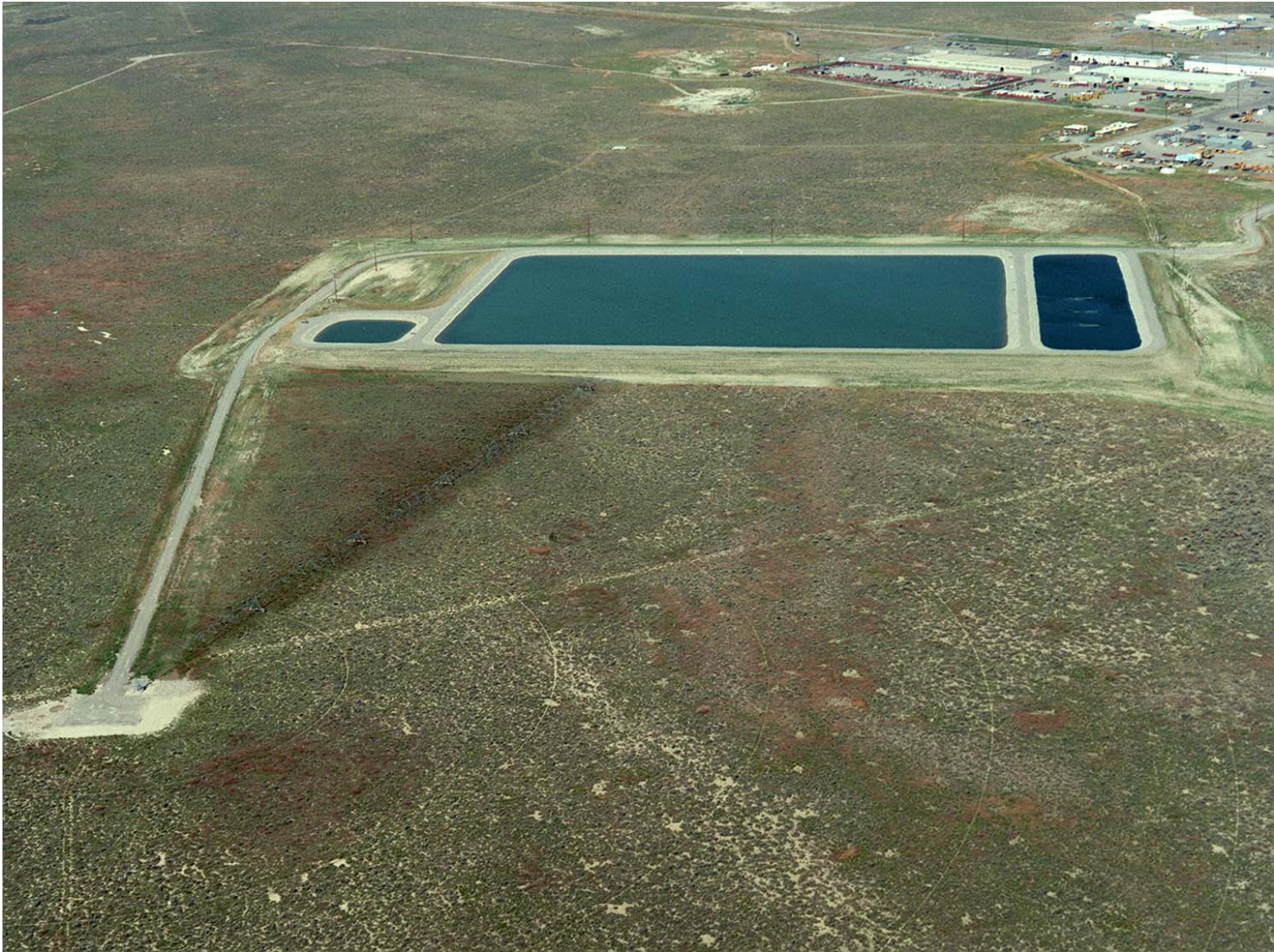
Figure A-1. Central Facilities Area Sewage Treatment Plant, 1995 (95-627-7-4).
