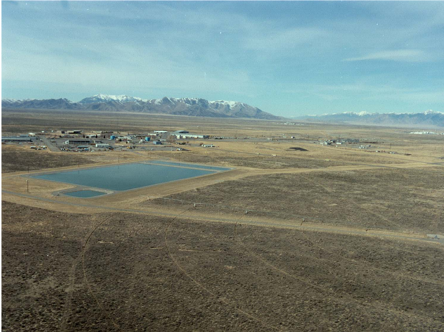
Figure A-2. Central Facilities Area Sewage Treatment Plant, 1996 (96-174-9-8).
