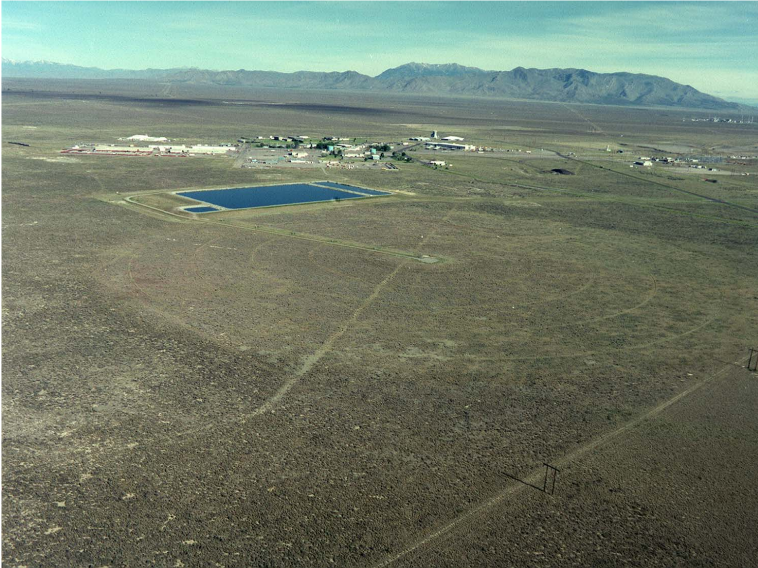
Figure A-6. Central Facilities Area Sewage Treatment Plant, 2000 (00-296-2-2).
