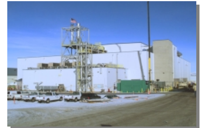
Construction was completed on Dec. 27, 2002 on the Advanced Mixed Waste Treatment Facility. Numerous facilities at the Radioactive Waste Management Complex were turned over to BNFL Inc. on Dec. 31, 2002.
