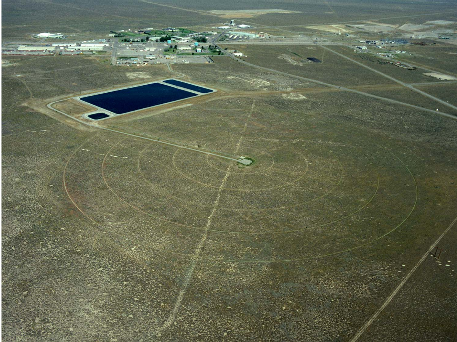
Figure A-3. Central Facilities Area Sewage Treatment Plant, 1997 (97-620-5-14).
