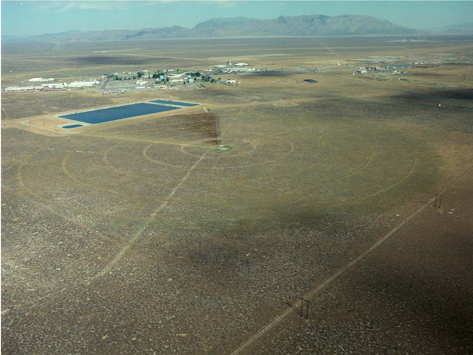
Figure A-4. Central Facilities Area Sewage Treatment Plant, 1998 (98-454-11-6).
