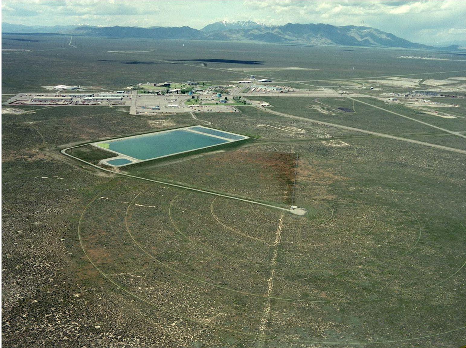
Figure A-5. Central Facilities Area Sewage Treatment Plant, 1999 (99-344-10-9).
