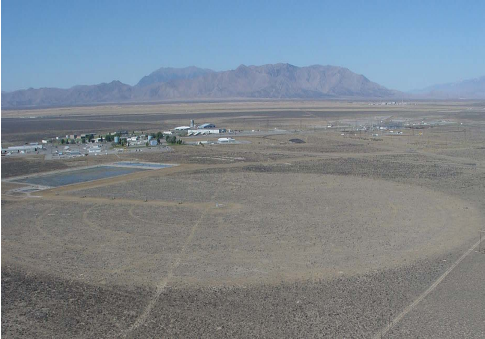
Figure A-8. Central Facilities Area Sewage Treatment Plant, 2003 (PD030339-01)
