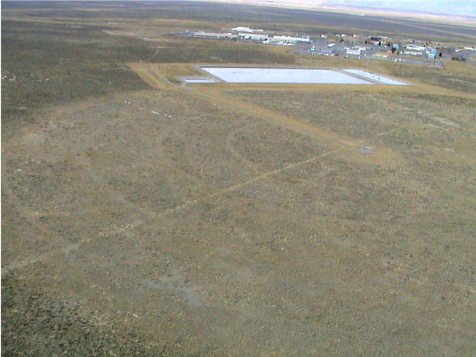
Figure A-7. Central Facilities Area Sewage Treatment Plant, 2002 (PD020741-02).
