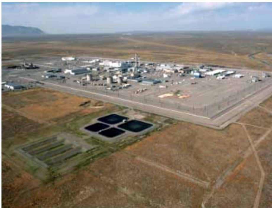
Figure B-2. Aerial view of the Idaho Nuclear Technology and Engineering Center.
