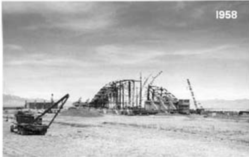
CONSTRUCTION OF HANGER AT TAN
