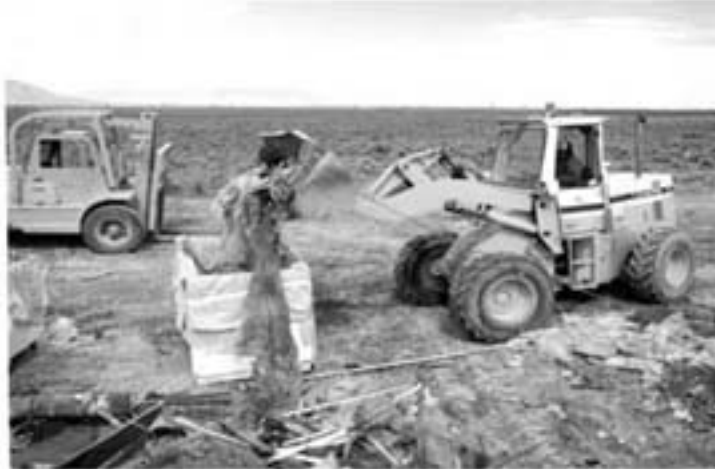
REMOVAL OF OLD TRASH DUMP DEBRIS AT BORAX
