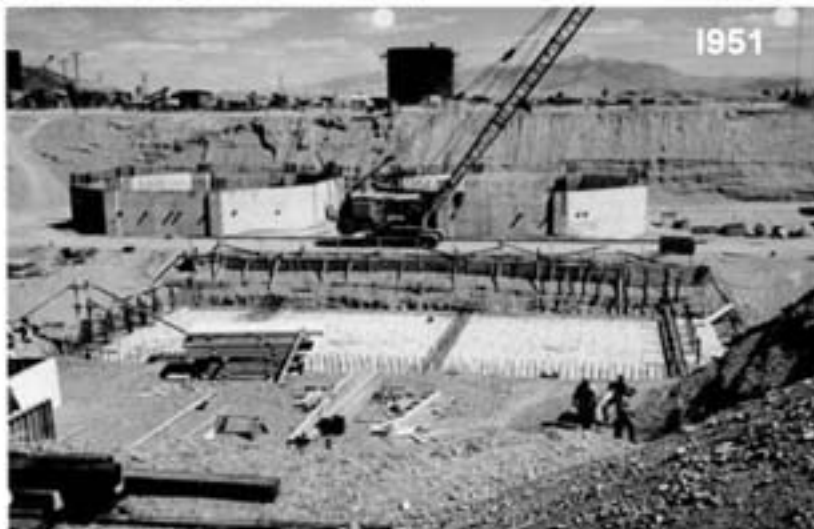
CONSTRUCTION OF TANK FARM AT INEEL
