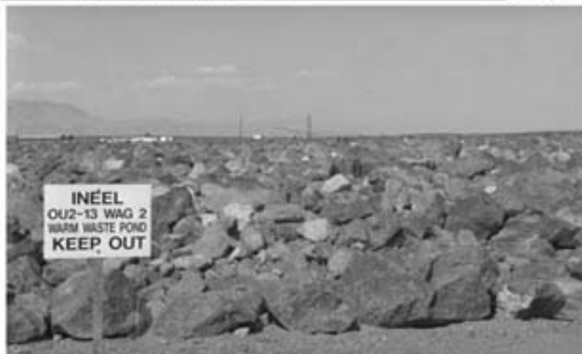
ROCK-ARMORED CAP ON REMEDIATED WASTE DISPOSAL POND AT TRA
