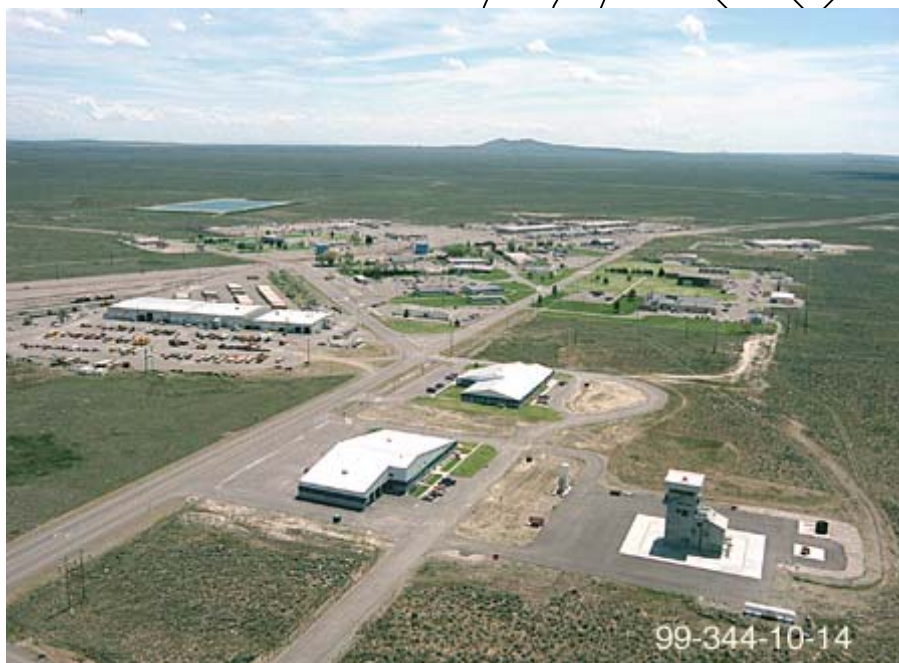
Figure 4-5. Aerial view of the Central Facilities Area.
