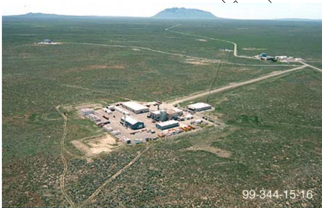
Figure 4-6. Aerial view of the Waste Experimental Reduction Facility with the Control Area shown in the distance.
