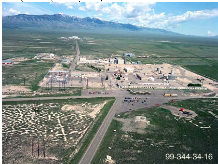
Figure 4-2. Aerial view of the Technical Support Facility at Test Area North with the Contained Test Facility in the background.
