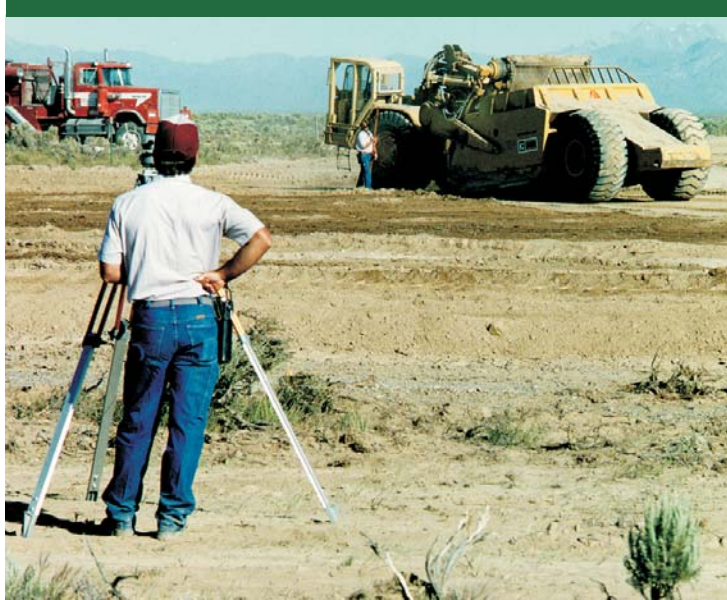
Surface contouring at the Subsurface Disposal Area.
