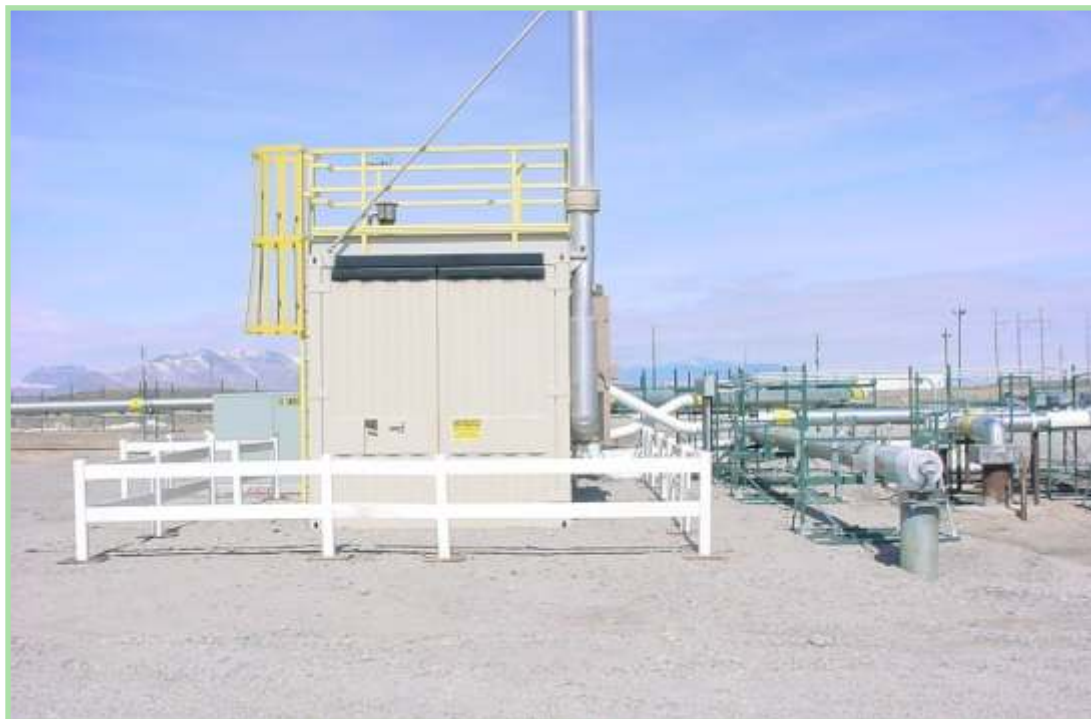
Vapor vacuum extraction units located in the Subsurface Disposal Area destroy harmful organic solvent vapors from the ground beneath the Radioactive Waste Management Complex.
